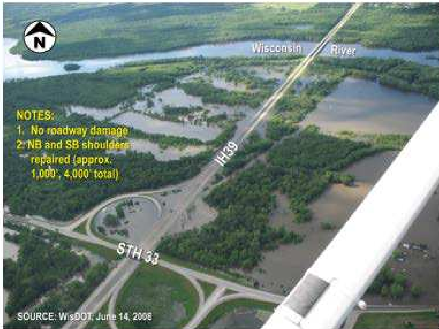
Aerial View of Extent of Flooding for IH39 at STH 33
