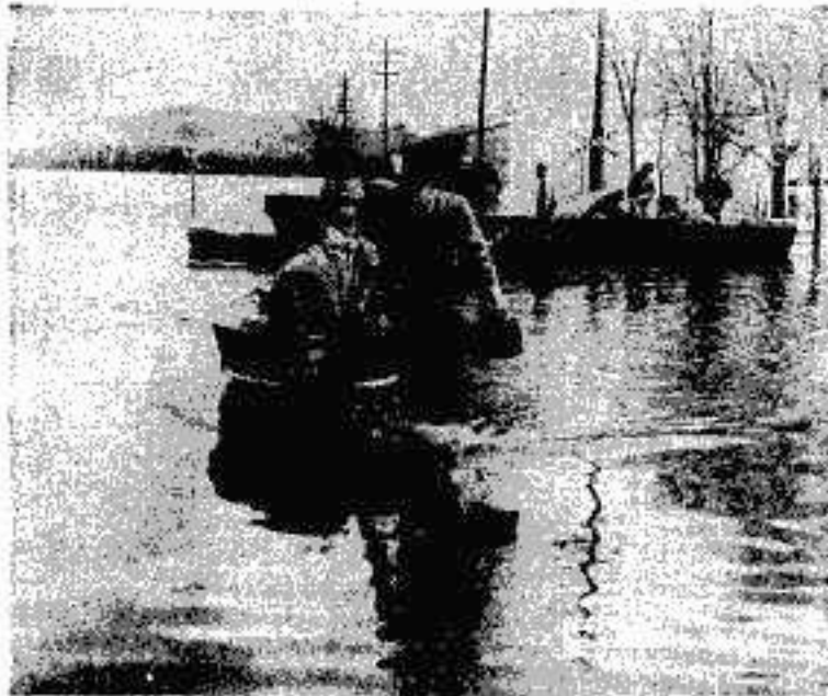
BOAT TRANSPORTATION . . . Employees of MSP are being transported to and from their Liberty street power station in boats. (Sunday News photo)
