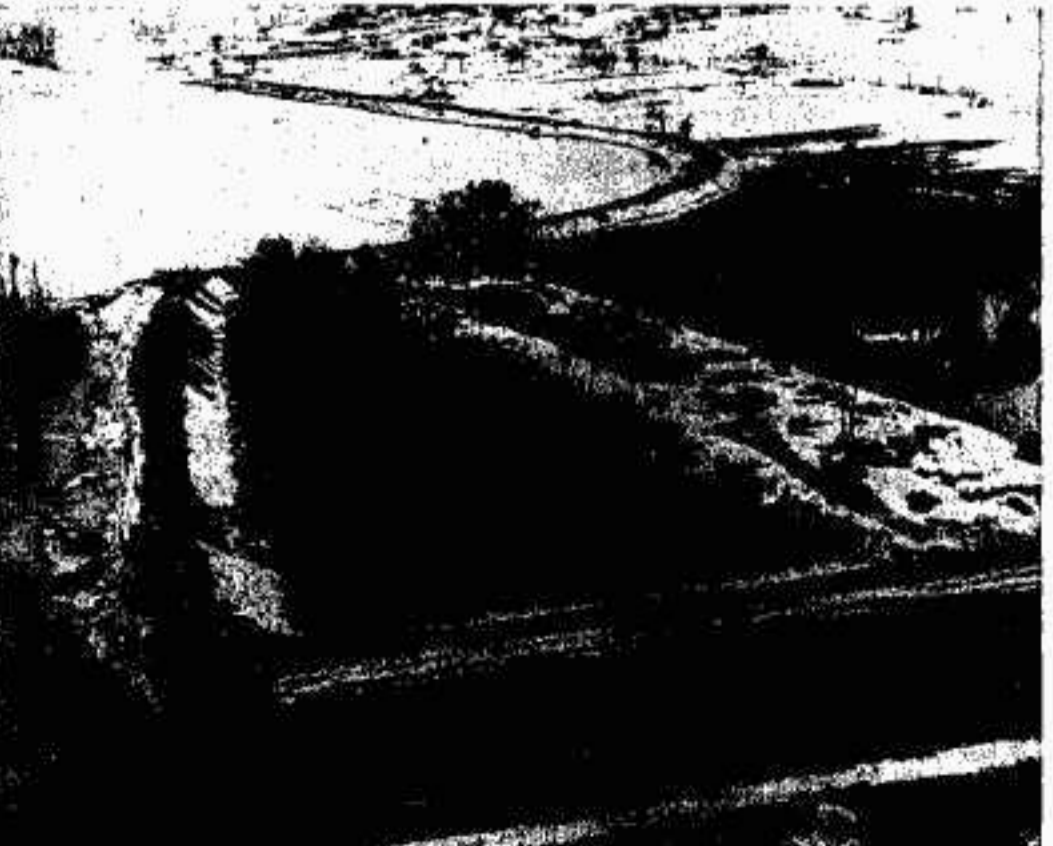
HEAVY ACTIVITY . . . The Muskoka Avenue area dike was being beefed up by dike workers Saturday noon. This air view, looking towards Highway 61 and Sugar Loaf, shows the dike now under construction. Patches of snow from Friday's snowfall remain on the ground. (Sunday News photo)
