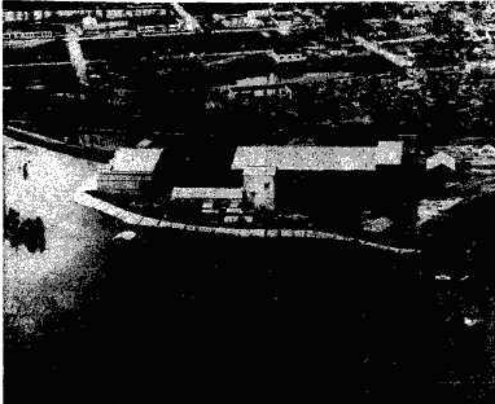
ARMOUR PLANT . . . Dikes still protect the Armour Agricultural Chemical Co. plant on East 4th Street today. The
