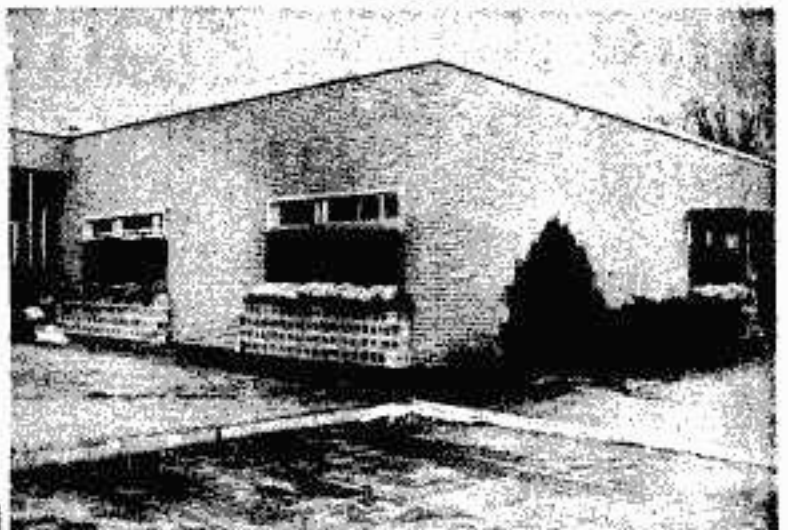
NEWSPAPER READY . . . Here's a view of a part of the Daily & Sunday News plant at 601 Franklin St. Obviously its ready to withstand some water. Inside structures have been prepared — should water get inside — to keep typesetting machines and other equipment dry. In event that the newspaper could not be published in this plant, it would be printed in Rochester. A few doors into the plant, including the Franklin Street entrance, remains unbaricaded at present. (Sunday News photo)
