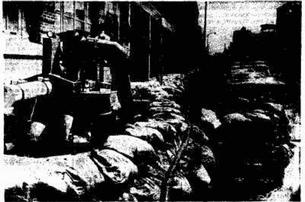
PROTECTING TELEPHONES . . . Looking east on 3rd Street from Johnson Street, the extensive pumping operation of the Northwestern Bell Telephone Co. Water is removed from the basement of the old and adjoining new structures.
