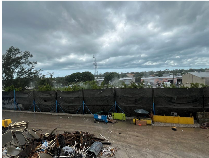
Figure 1: SW view of misters on West Perimeter fencing
