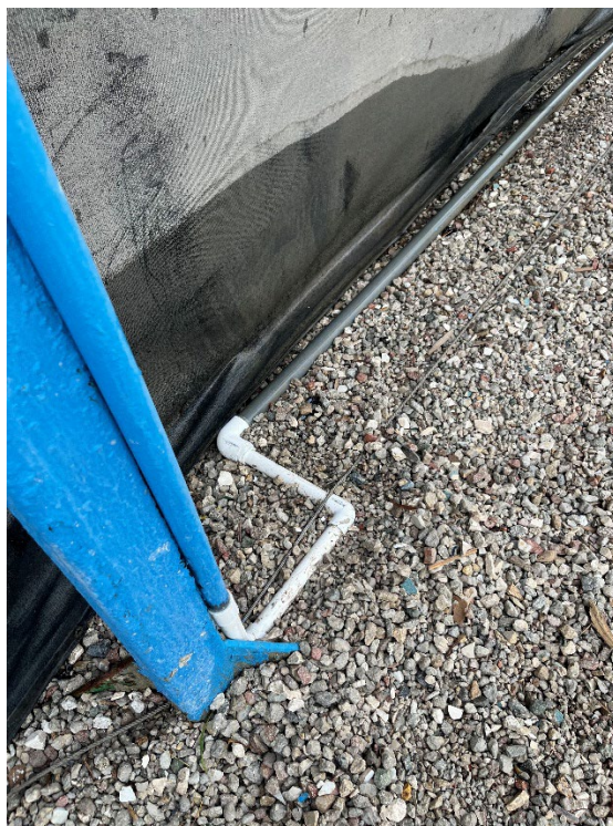
Figure 4: View of repaired pipe connection that feeds water to the misters
