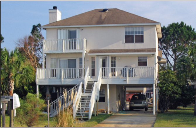
Elevated home on pile foundation
