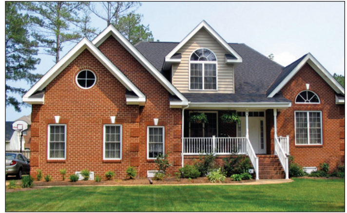
Elevated home on crawl space foundation
