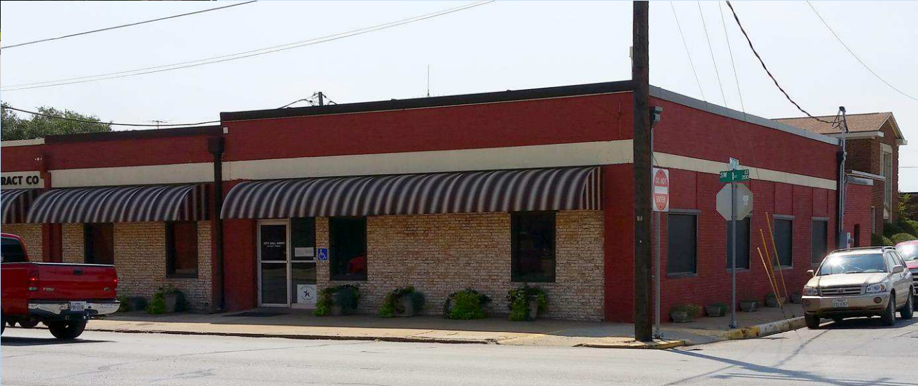
City Hall Annex
