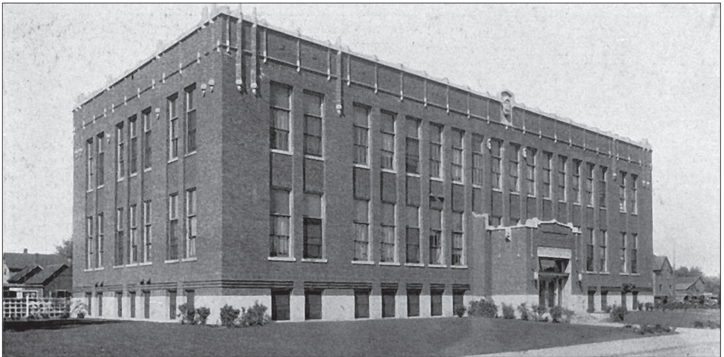
The Rath Administration Building, c. 1925.
