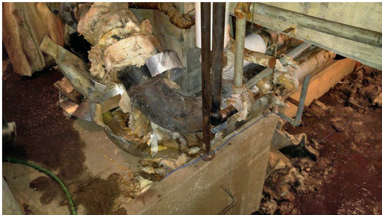
Figure 1: Area where wet insulation was found at the south end of the utility tunnel. (The insulation was removed from the elbow as part of the investigation.)
