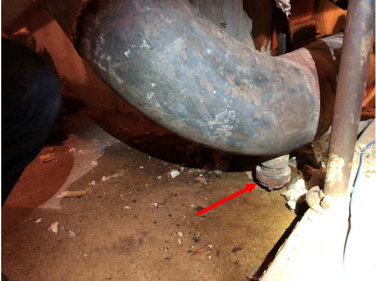
Figure 2: The location of the 2" drain and the failed cap. (All insulation has been removed as part of the investigation.)
