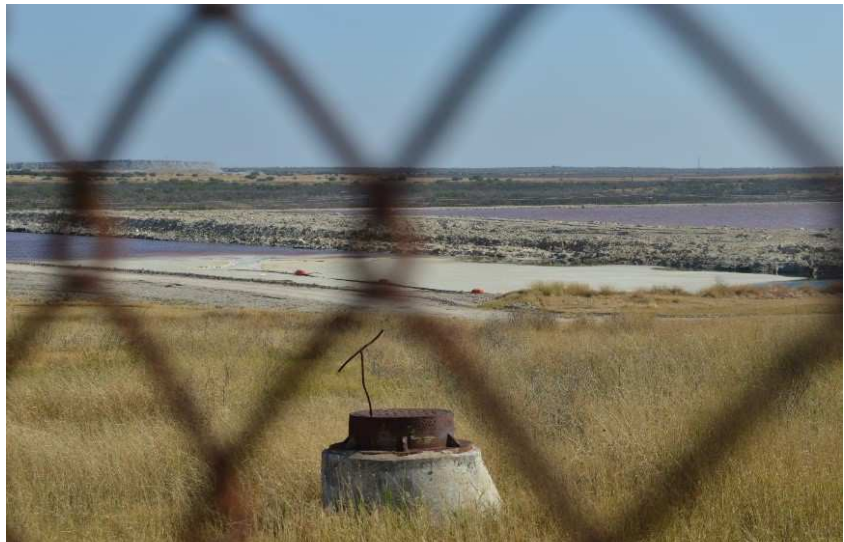
Behind this fence is the coal ash pond near the Peeler ranch that is leaking contaminants into the groundwater.
