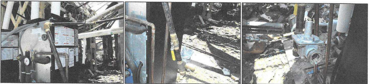
Figure 26: The natural gas line supplying the north and south water heater units were disconnected and the ball valves were in the open position.
