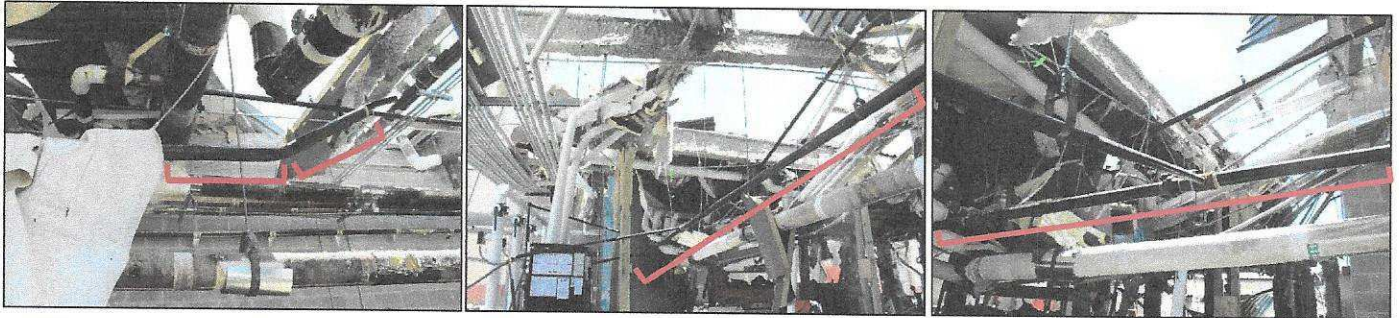
Figure 25: A riser extended from the "tee" on the roof to the mechanical room. A horizontal pipe then supplied natural gas to each water heater.
