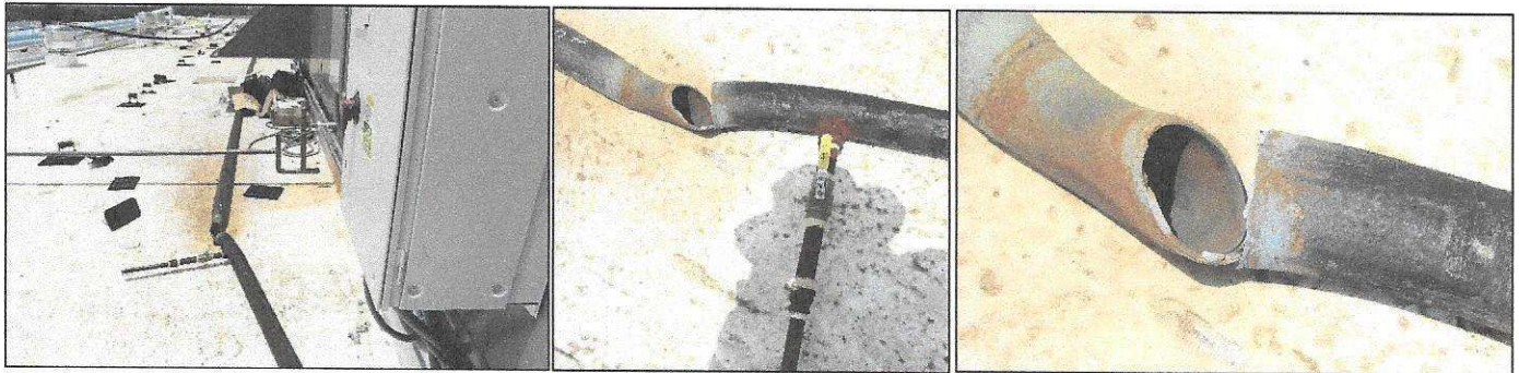
Figure 14: The natural gas line has dislodged from its support structures (black pads and rooftop rollers); fracture at a welded 90° elbow.
