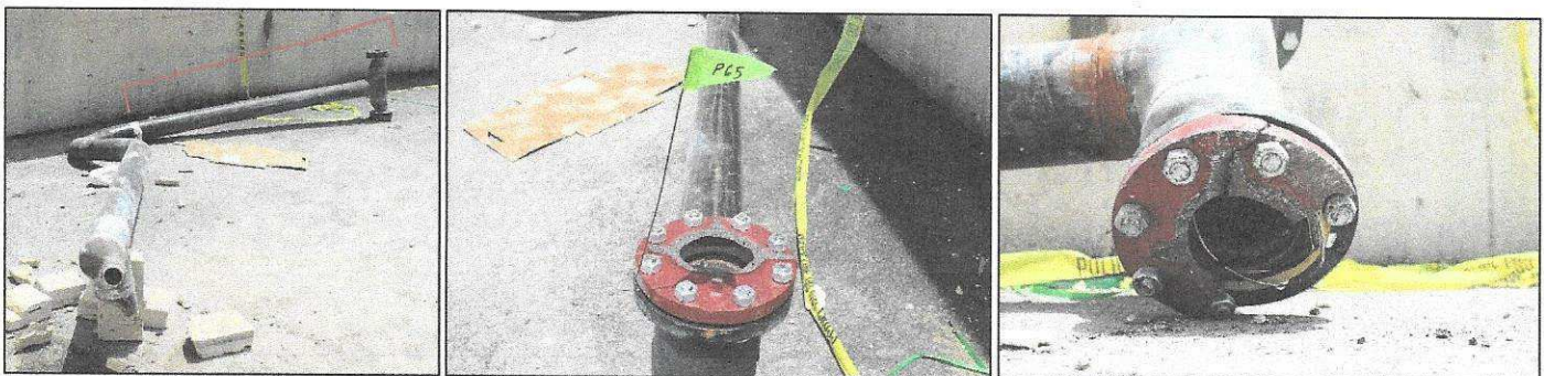
Figure 21: One side of the "tee" extended to the boiler room. The section above (marked in red) was identified as the riser to the boiler room. A "tee" was welded at the end of the riser with a fractured flange on each side of the "tee."
