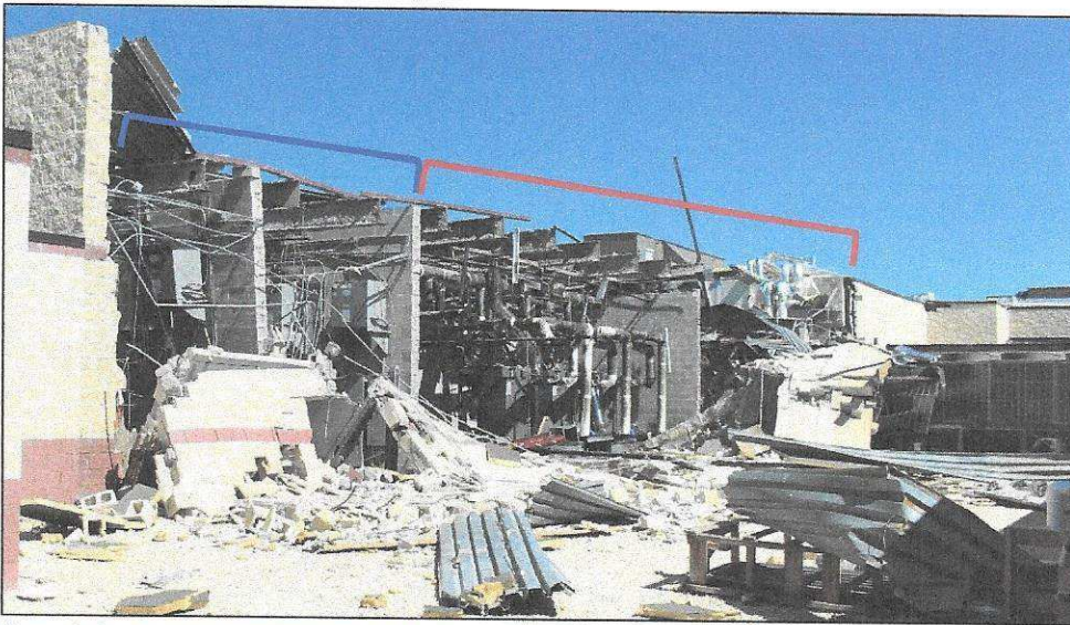
Figure 8: Damage to Western Wall of Mechanical, Boiler, and Electrical Rooms
