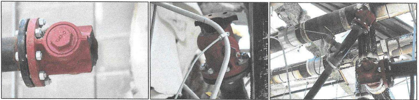
Figure 22: The fractured flanges shown in Figure 21 matched the fractured cast iron plug valve housings in the boiler room.
