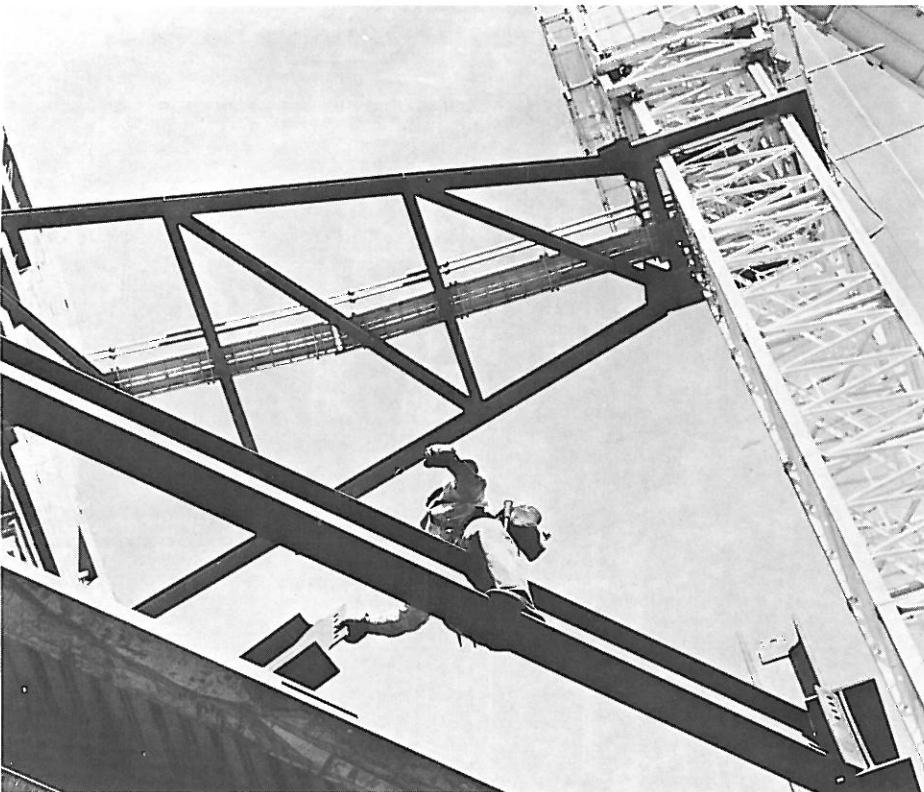
Currently workers are erecting the structural steel framework for the building.
