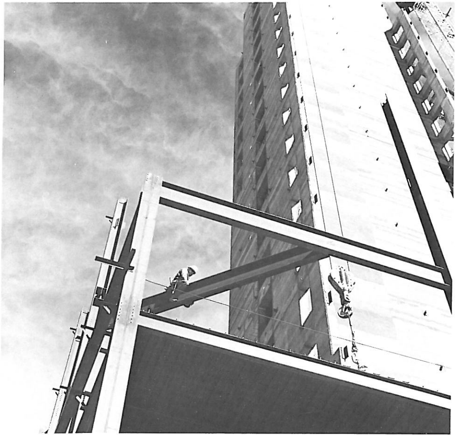
Some 330 tons of reinforcing steel was used in the core.
