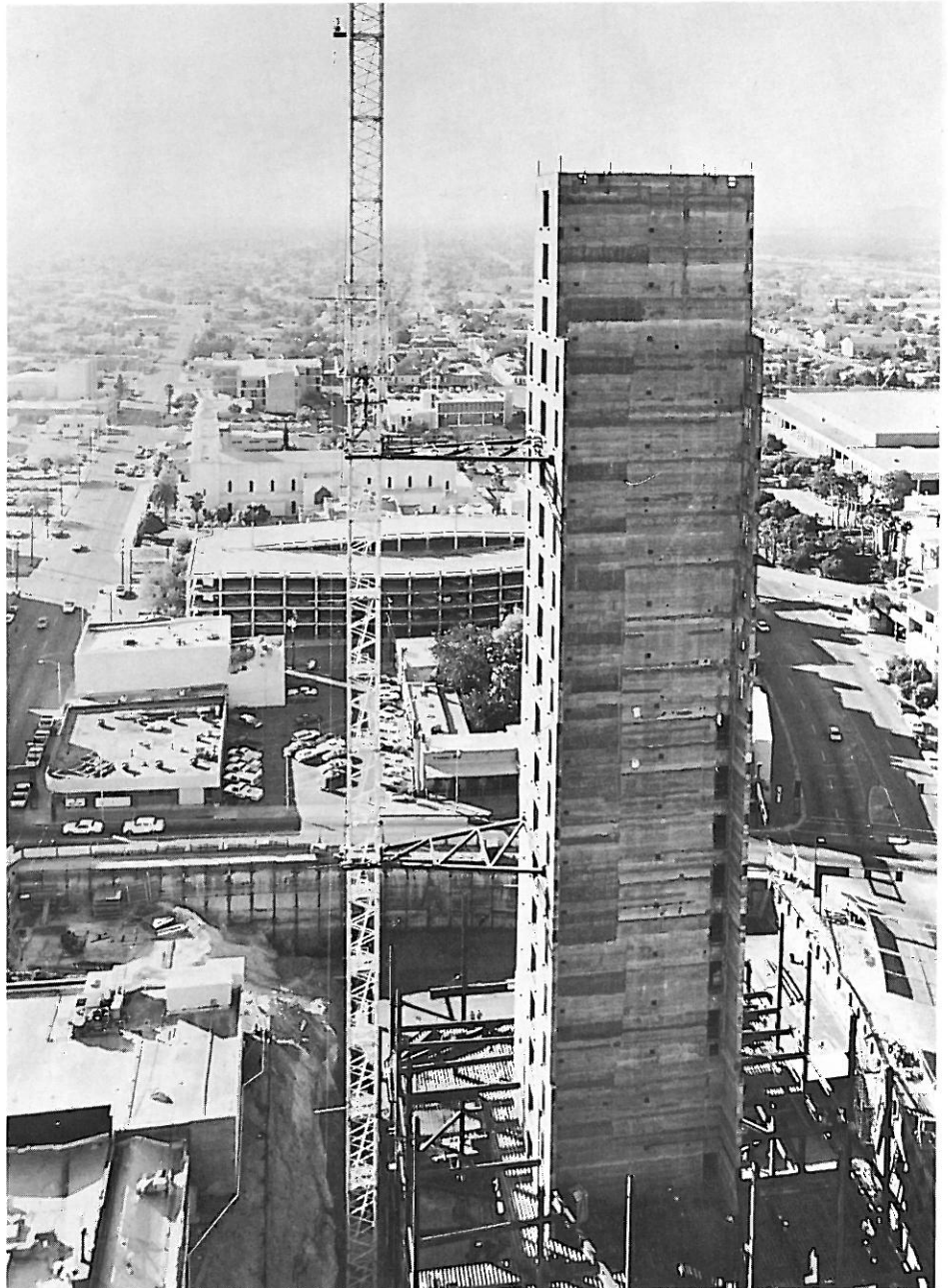
Slipforming the tower's core took approximately one month and used a total of 2,400 cubic yards of concrete.
