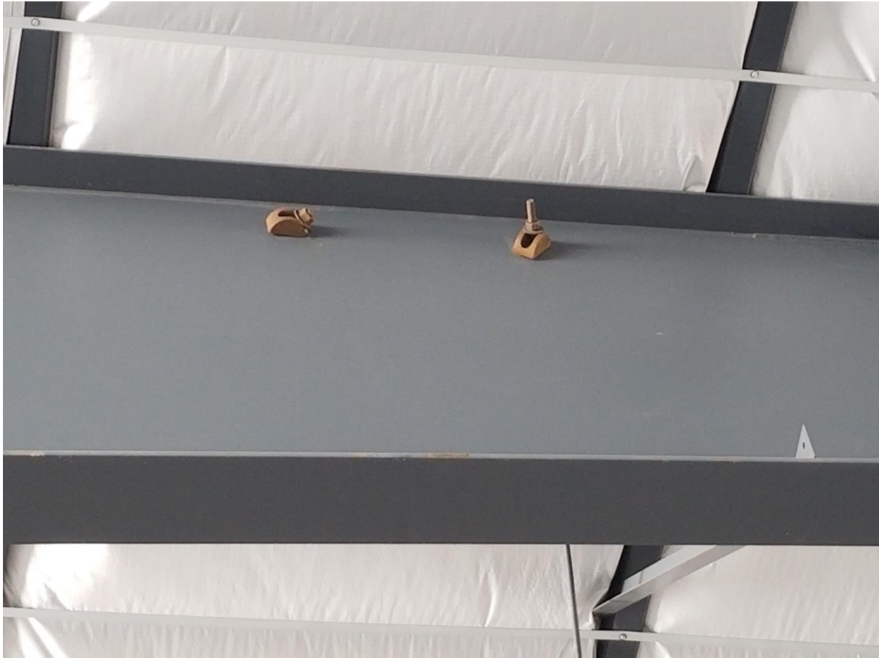
Photo #5 – More hillside washers displaced
