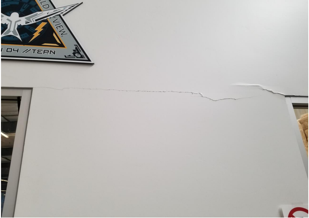
Photo #3 – Crack in observation wall failure
