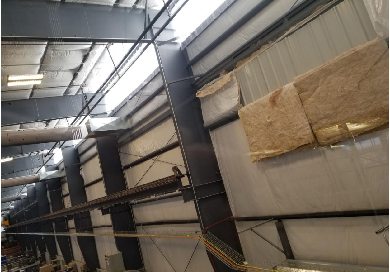
Photo #4 - Damage in high bay area showing girt damage
