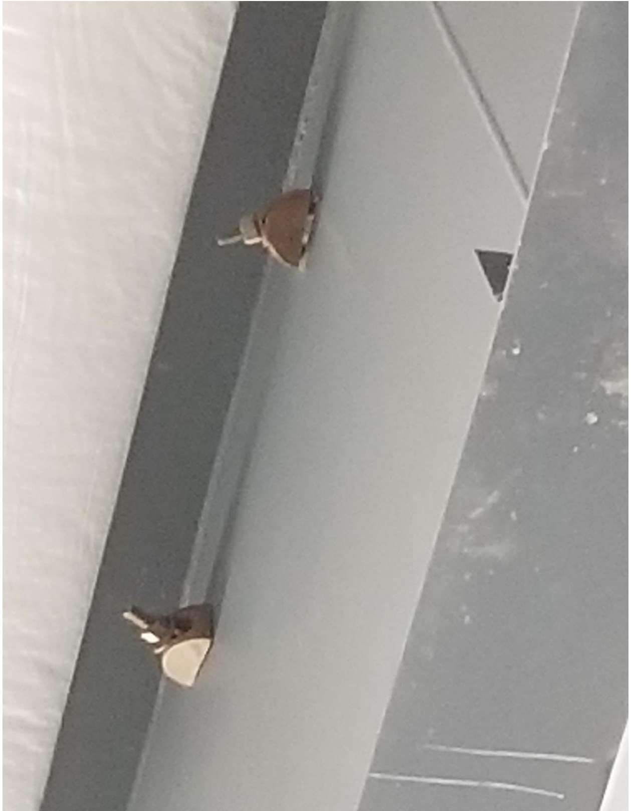
Photo #1 – Hillside washer displaced
