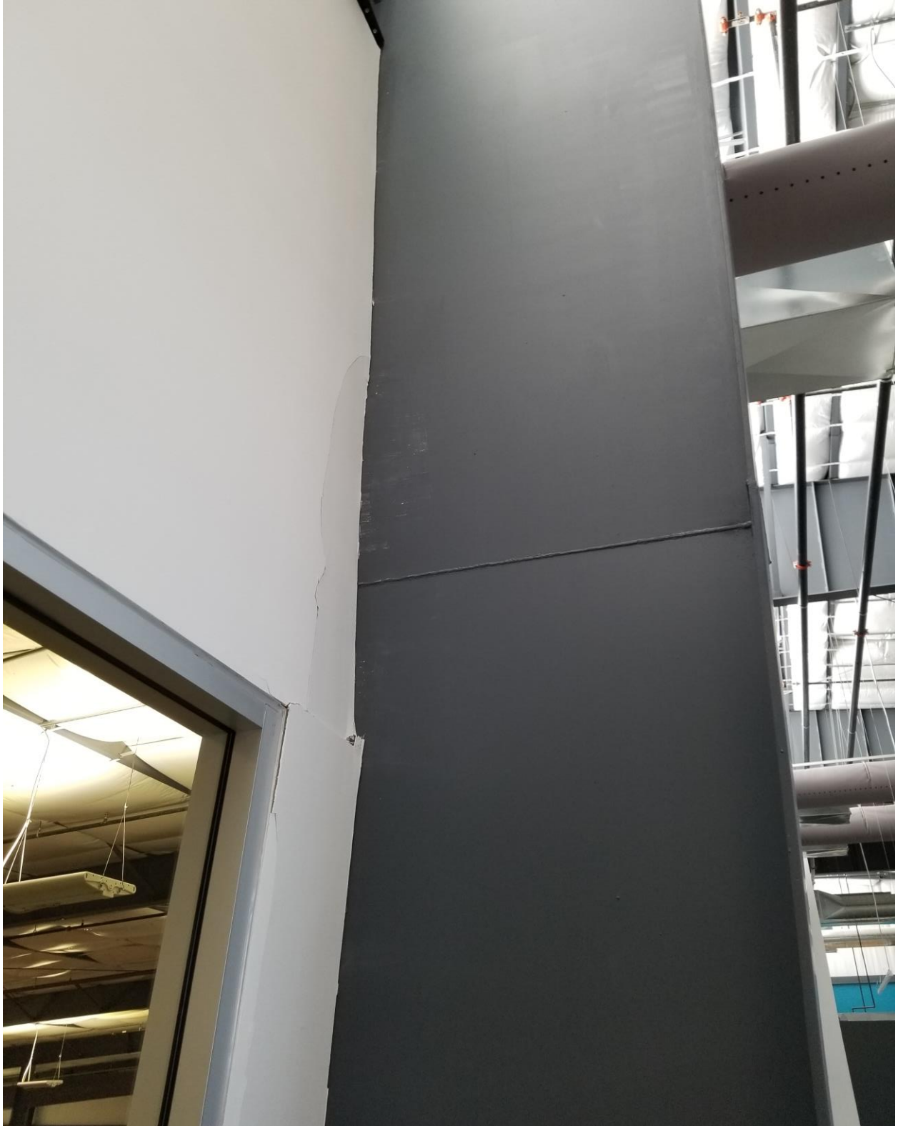
Photo #2 – Interior non-bearing wall failure with marks on column showing amount of movement experienced.
