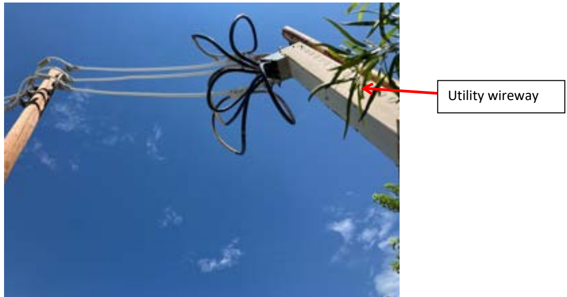
Figure 1. Overhead Utility lateral serving Mobile Home Park.
