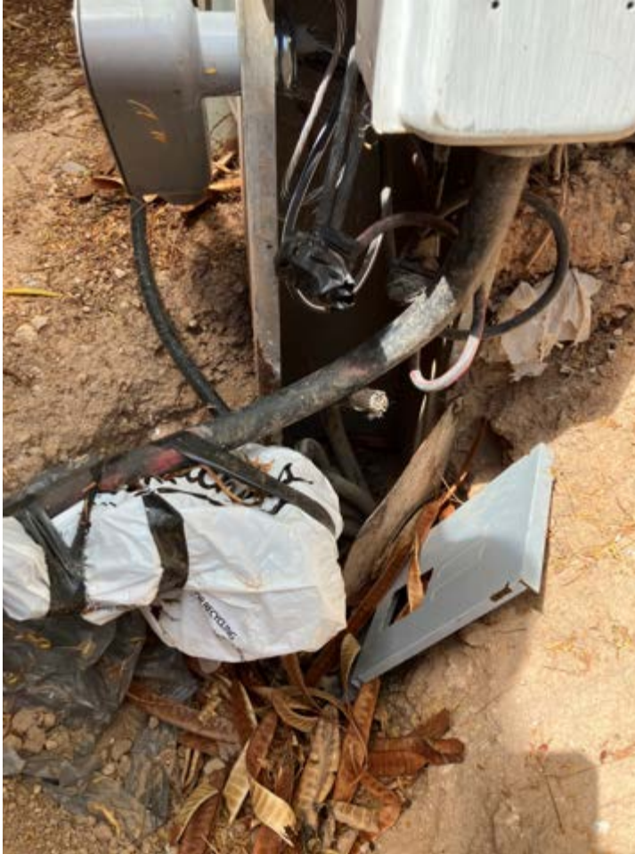
Figure 7. Temporary power feed into pedestal.
