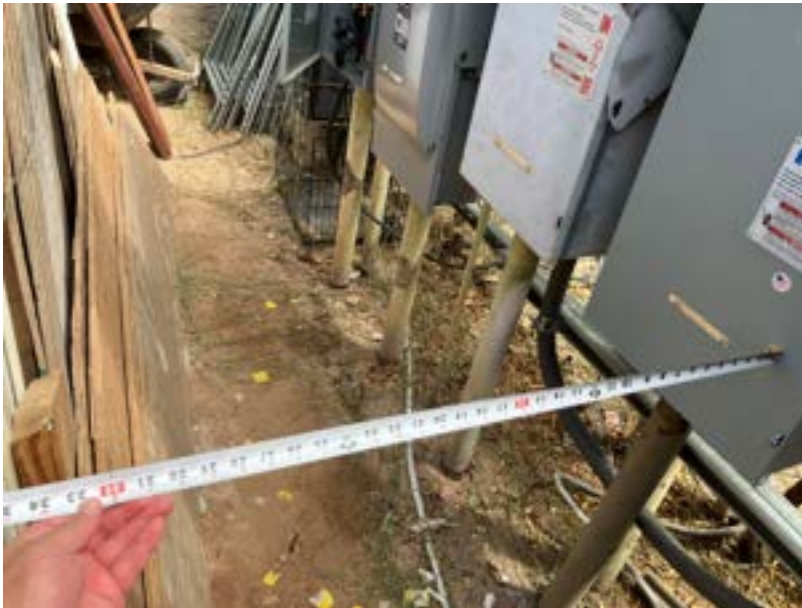
Figure 9. Tape measure showing less than approximately 30 inches of horizontal clearance in front of the disconnect switch panels.
