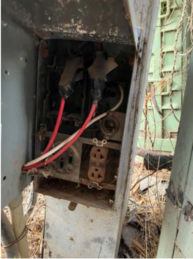
Figure 8. Conductors running outside the envelope of the pedestal enclosure.
