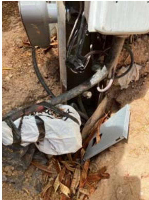
Figure 4. Temporary power feed into pedestal.
