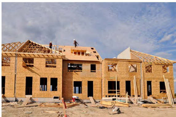
Construction in Marana. Source: Town of Marana
