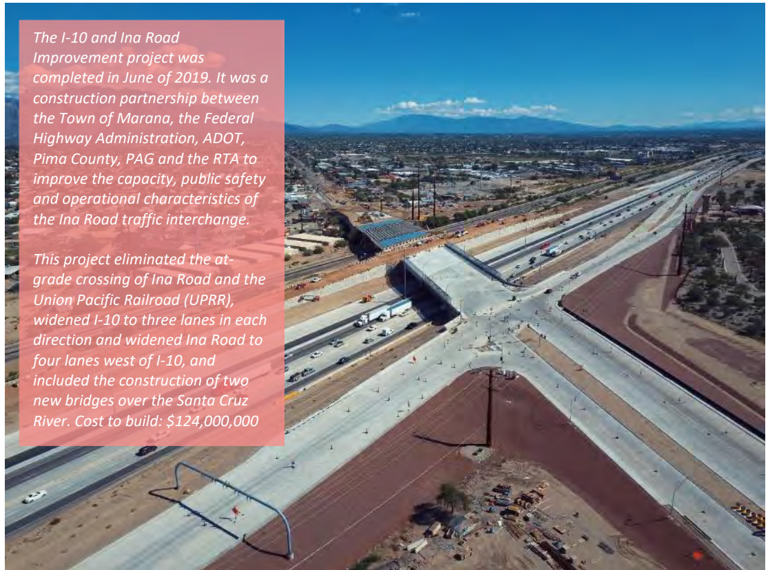
Ina Road construction. Source: Psomas
