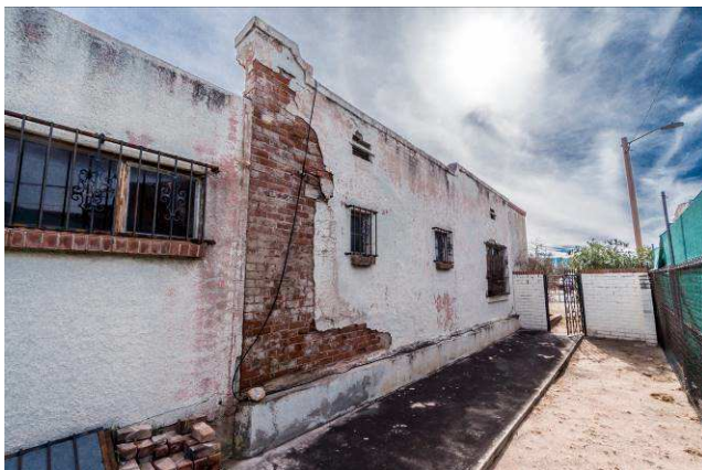
Exposed Brick and encapsulated stone foundation
