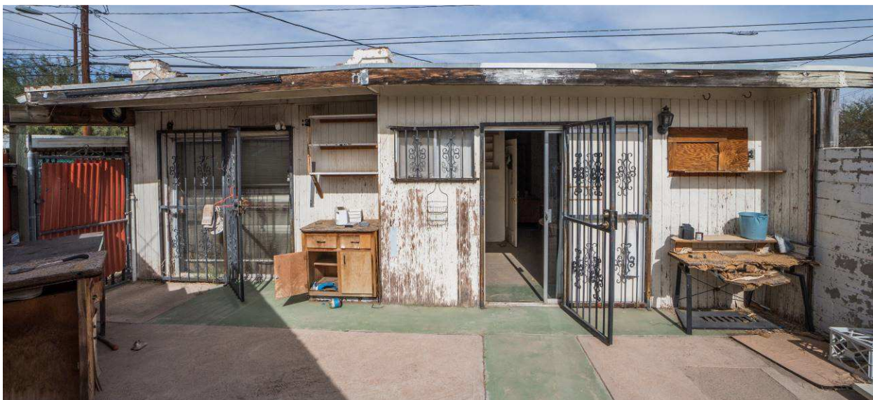
Outbuilding South Facade
