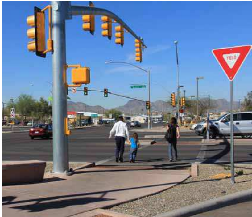
Indirect left turn at Grant and Oracle. Well-signed “porkchop” and pedestrian islands break up crossing. Eliminating left-turns on Grant reduces potential conflicts.
