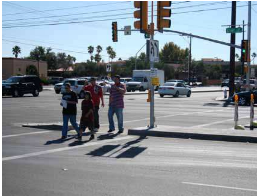
Accessible pedestrian refuge island with push button signal activation for pedestrians who are unable to cross the roadway in a single phase.
