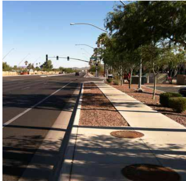
A shaded sidewalk with buffering improves pedestrian comfort on this suburban arterial street. Image: Town of Marana
