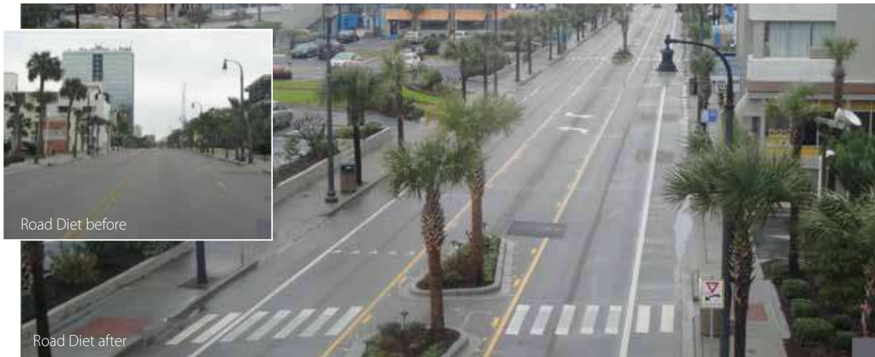
Example of a four to three lane road diet in Myrtle Beach, South Carolina. Five lanes of traffic were converted to two travel lanes, a center turn lane and bike lanes. The addition of landscaped median islands and high visibility crosswalks improves pedestrian safety and provides more crossing opportunities. Image 1: Google. Image 2: City of Myrtle Beach. Road diet example from rethinkingstreets.com
