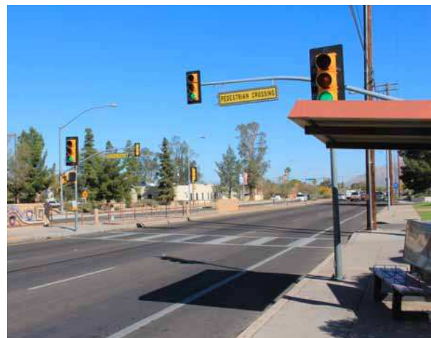
Pedestrian island with staggered high-visibility crosswalk. The direction of the crosswalk goes against traffic for improved safety
