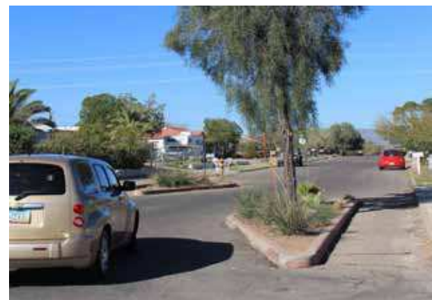
Example of a landscaped chicane on a residential street. The chicane diverts the direction of travel and slows speeds.
