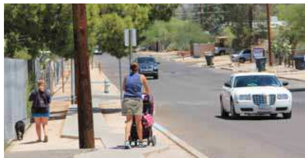
Continuous sidewalk on residential street segment. Utility conflict prevents installing a direct route but adequate right-of-way allows installation around barriers.
