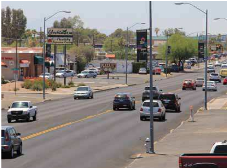
Busy four-lane arterial street in midtown Tucson. Multiple driveway cuts, sidewalk gaps and lack of shade make this a difficult walking environment. Pedestrian improvements are planned for this area.
