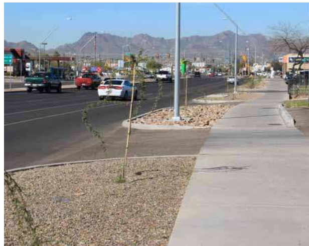
Wide sidewalks installed on newly improved urban arterial roadway. A 12-foot landscaping strip, continuous level 8-foot sidewalks, 11-foot travel lanes, and future tree growth in the planting strip make this a high-quality arterial pedestrian facility.
