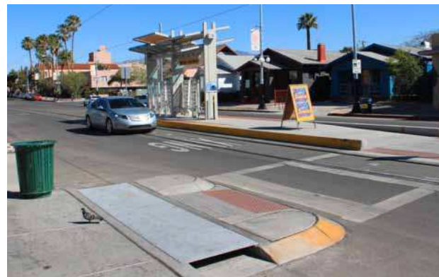
Mid-block curb extension at Tucson Modern Streetcar stop.
