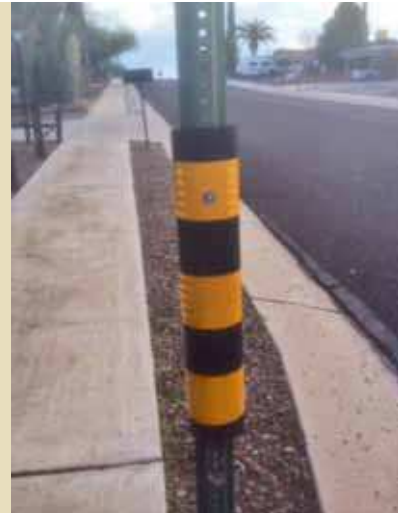
Example of plastic tubing on a road sign. Extending the tubing to the ground and potentially changing the coloring will distinguish bus stops from other types of road signs.
