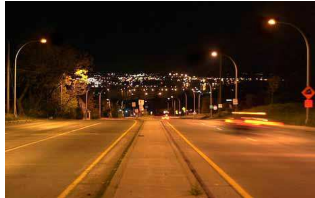
Staggered streetlights in Duluth, Minn., providing continuous arterial lighting. These lights feature full cut-off luminaires to reduce light pollution. Photo: Bob King
