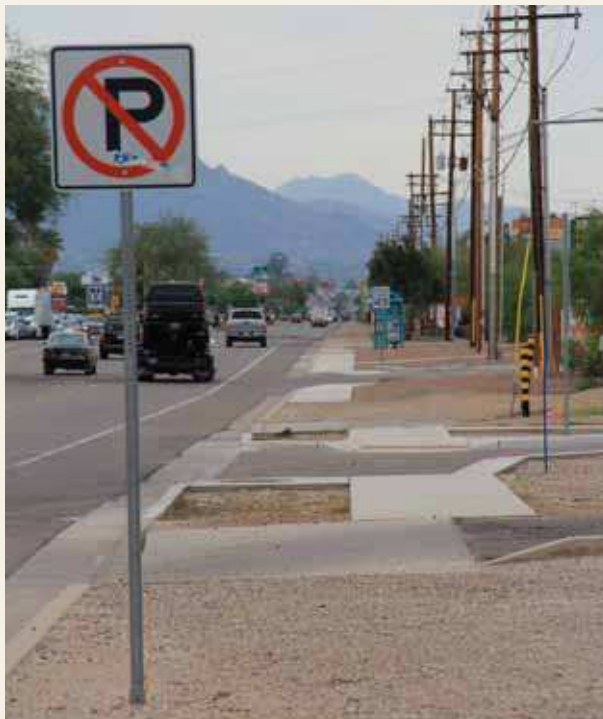
Sidewalk gaps such as this are seen throughout the region.
