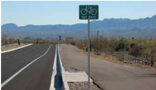
Shared-use path adjacent to roadway can accommodate both pedestrians and cyclists for a safe and comfortable travel and recreation option in a low-density location. Image: Town of Marana
