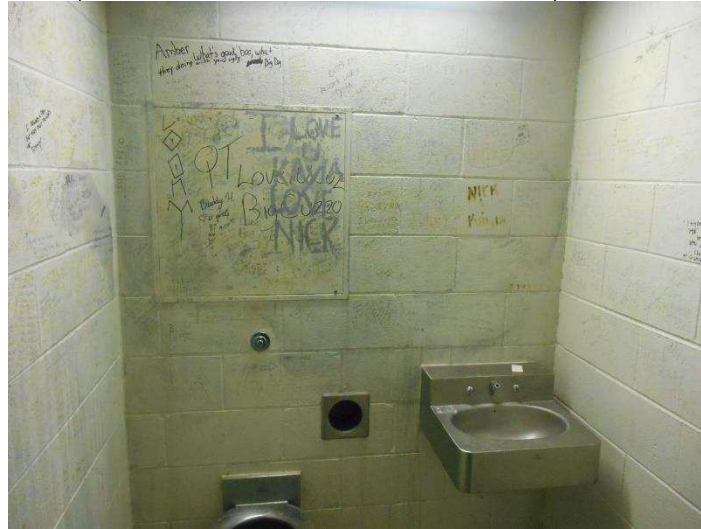
Figure 65: Inmate Bathroom on Top Floor New Side (Classrooms, Indoor/Outdoor Recreation)
