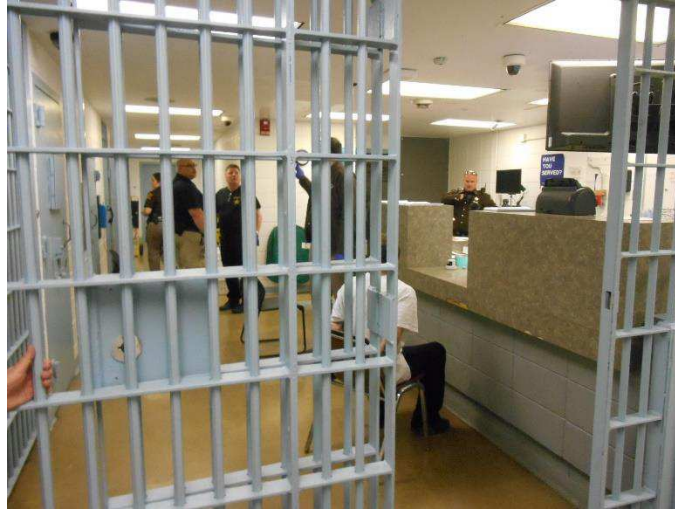
Figure 67: Intake Processing Area, Old Side, First Floor
