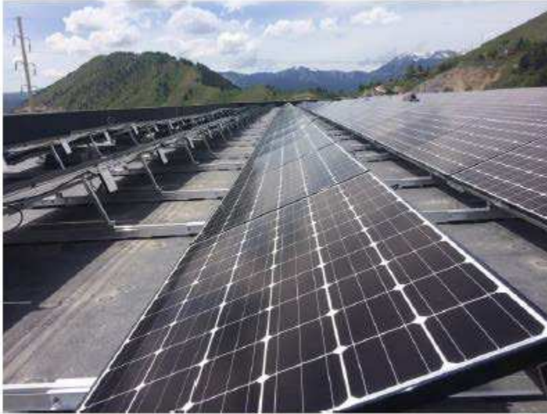
Figure 6 shows a solar generation facility built at the Integrated Solid Waste and Recycling Center in Teton County (Bruderer, et al. 2017).
