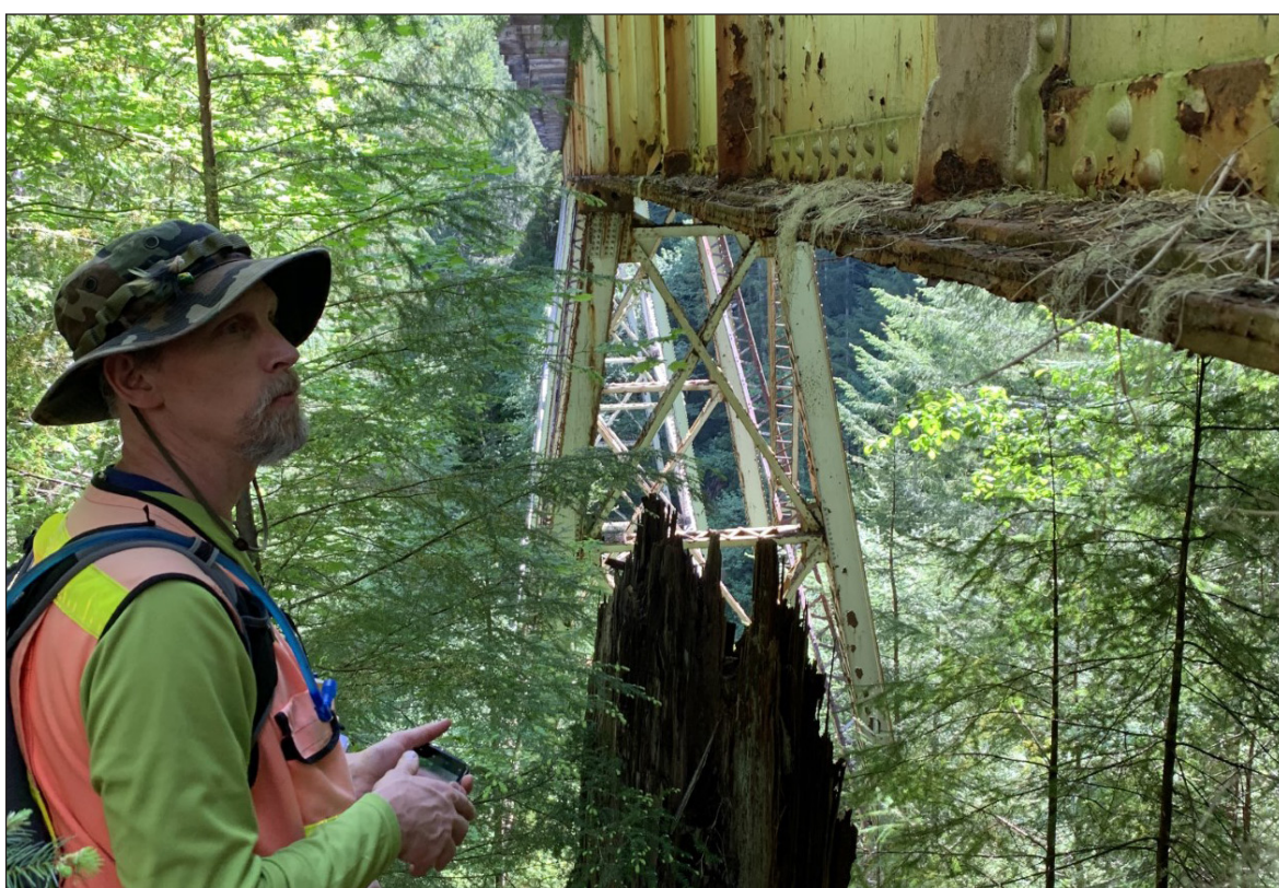
An engineer working where the rail line passes through the Tillamook State Forest. Photos Courtesy of Jon-Paul Bowles
