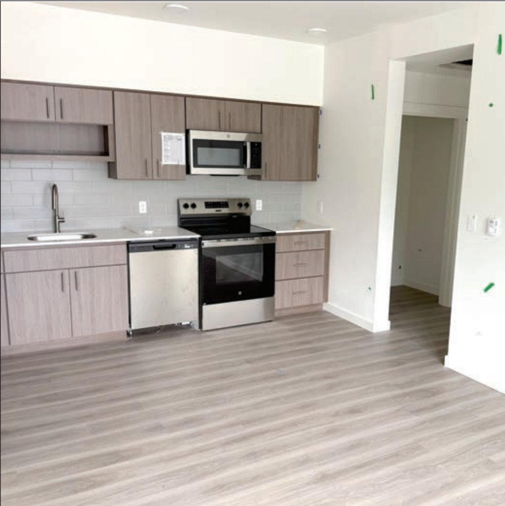
The kitchen in one of the more-complete apartments, featuring stainless-steel appliances and subway tile backsplash.
