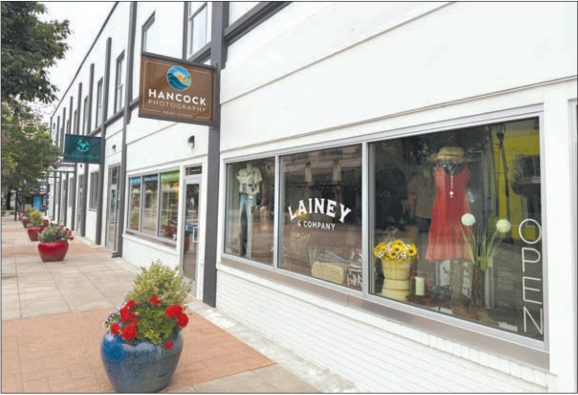
The remodeled national bank building’s downstairs retail spaces fronting on Henson Plaza.
