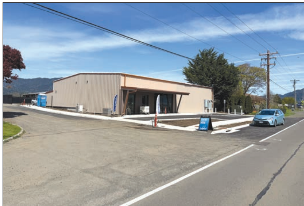
The center for industrial technology also underwent a recent renovation, with its exterior updated to tie in with the rest of the college.
