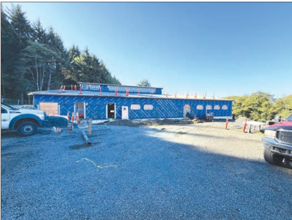
Work at the police station is ahead of the city hall, with a vapor barrier already installed in mid-October.
