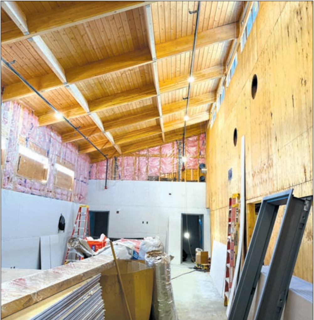
The area that will house the bullpen at the new police station.
