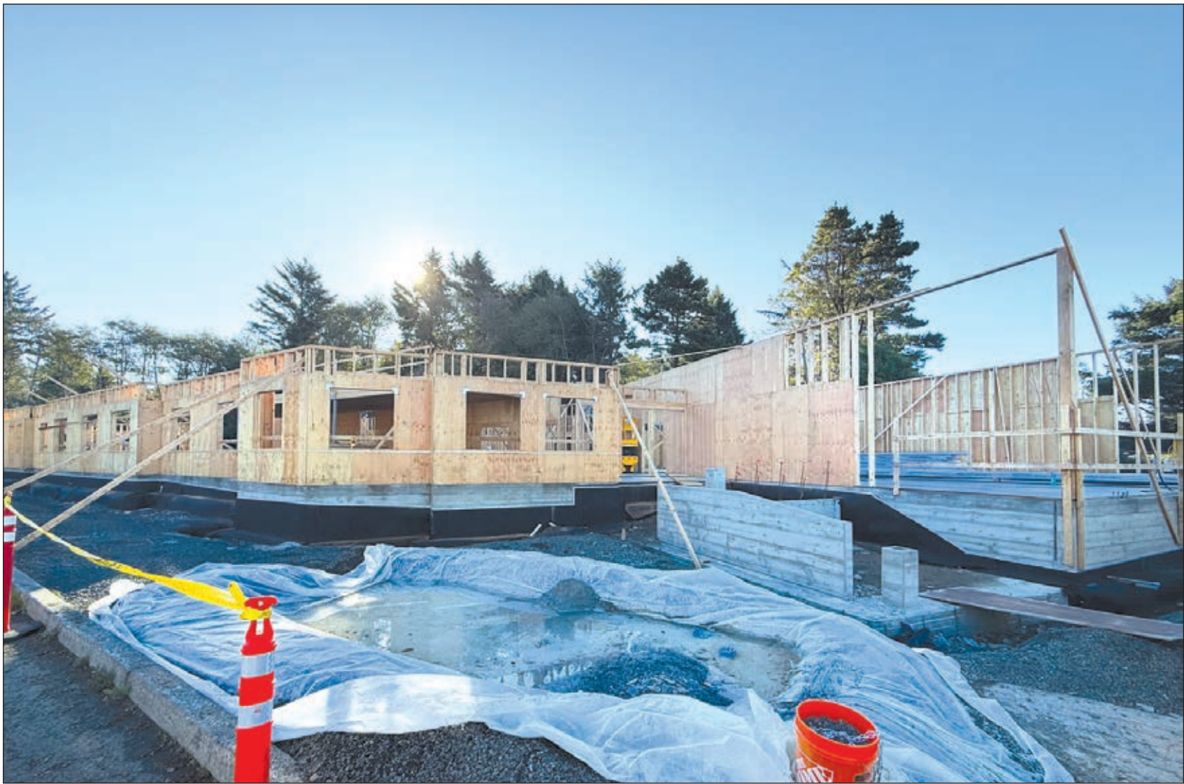
The new city hall's exterior as walls go up.
