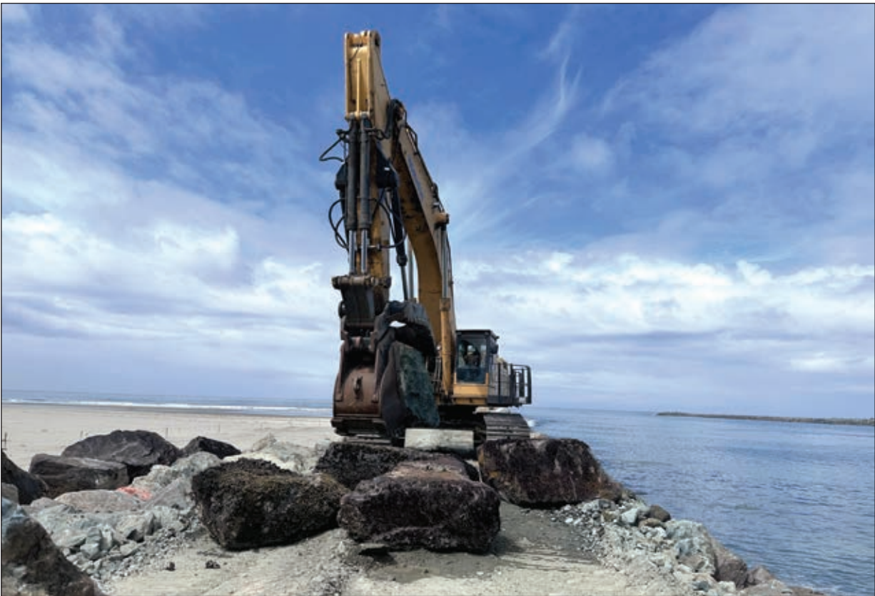
WILL CHAPPELL / COUNTRY MEDIA, INC. The excavator moves a legacy stone from the jetty’s original construction. Some of these stones are being moved to make place for new stones, but they will all end up back in the jetty, usually near their original location.
