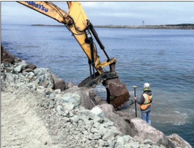
WILL CHAPPELL / COUNTRY MEDIA, INC. The stone placement team's spotter inspects the excavator's placement of a stone, prepared to log its location with a GPS beacon.
