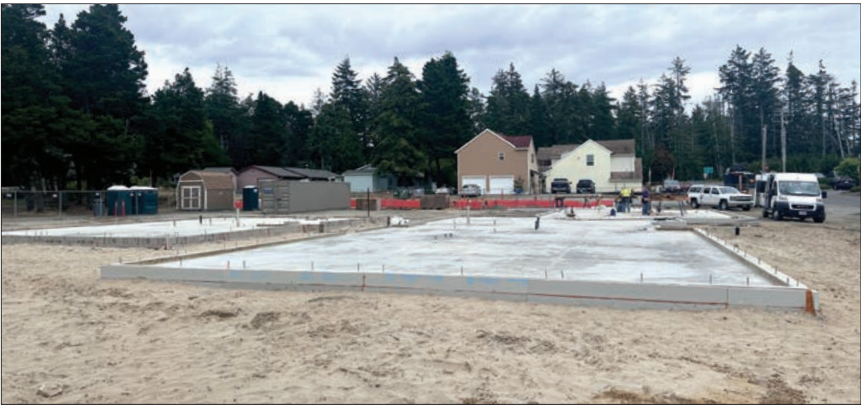
WILL CHAPPELL / COUNTRY MEDIA, INC. The concrete pads that will serve as the foundation for Manzanita’s new city hall and police station as seen from the west end of the property.
