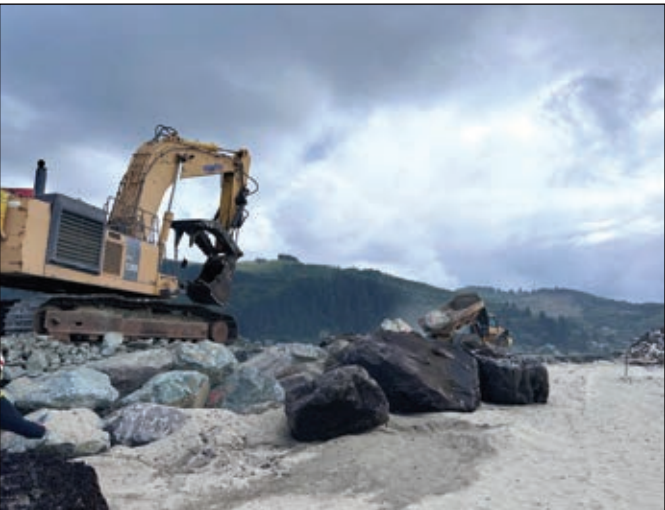
WILL CHAPPELL / COUNTRY MEDIA, INC. A transport truck dumps three stones on top of the jetty for the waiting excavator to place.
