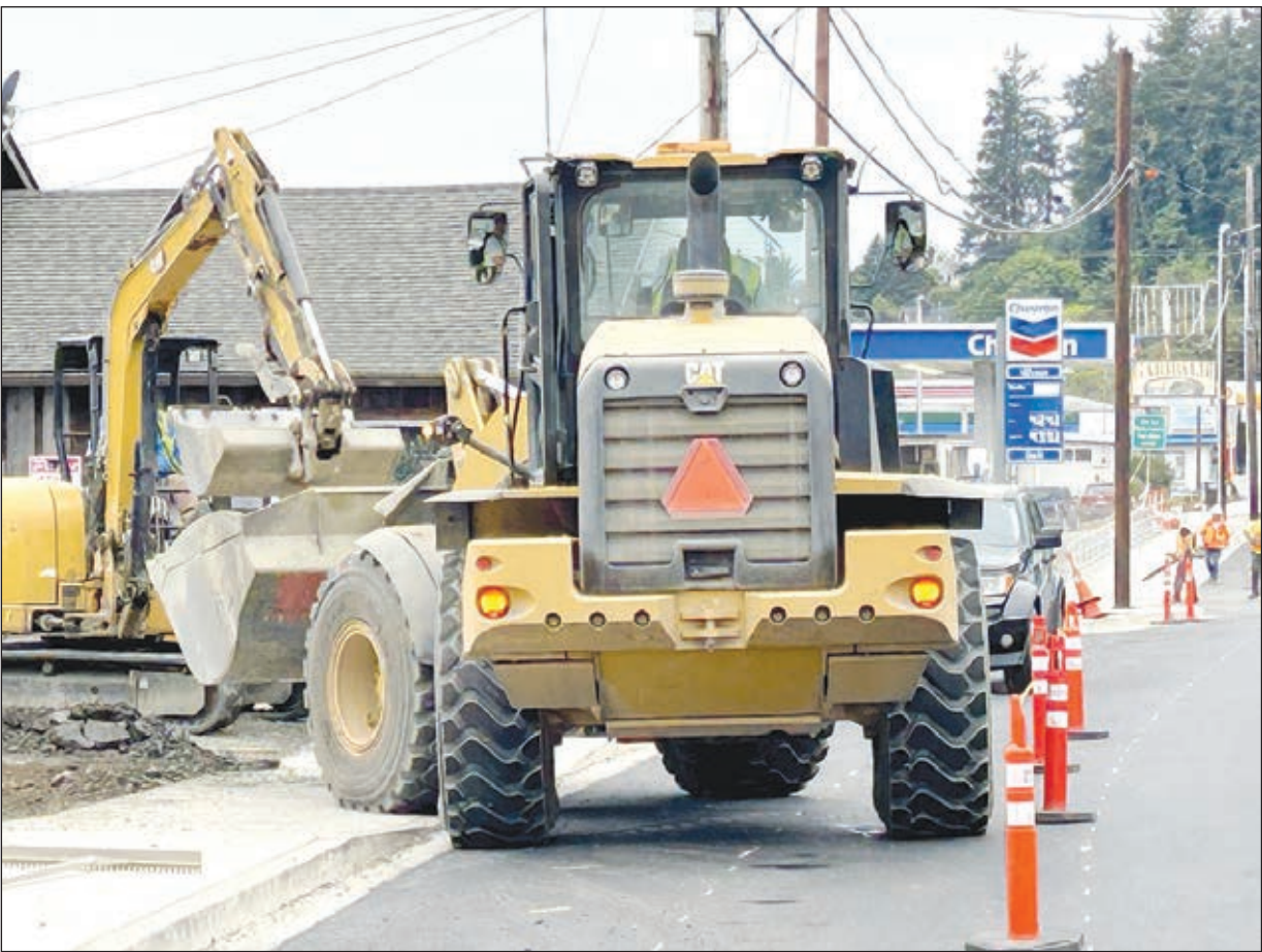
Workers making progress on the final touches of the highway upgrade project in mid-July. Photo by Katherine Mace
