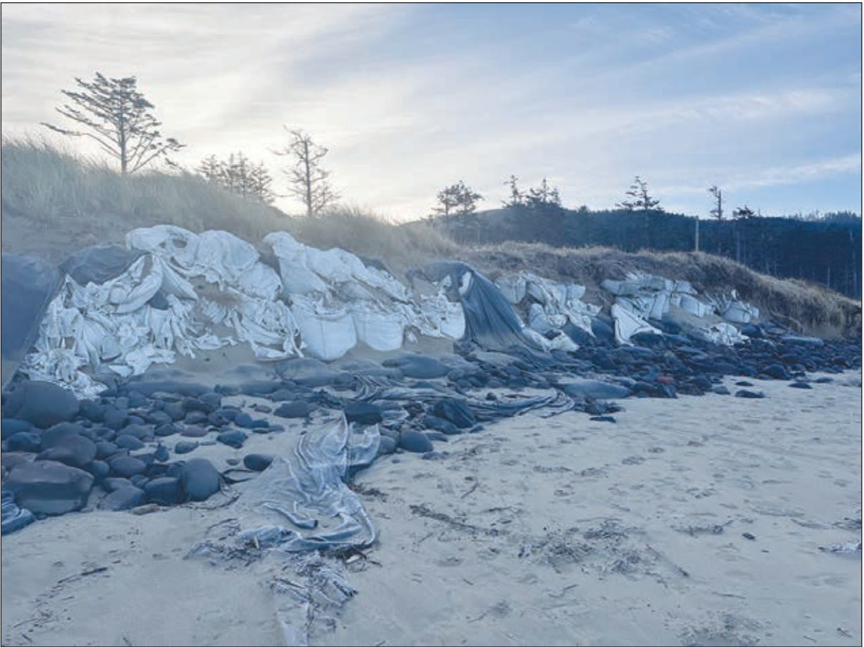
Photos by Will Chappell (Top) The section of the manmade dune at Cape Lookout State Park that has experienced the most sloughing because of wave and storm action and that will be repaired as part of the coming work. (Bottom) A view towards Cape Lookout with still-intact dune on the left.
