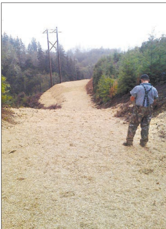
This highly important access road to the power poles is a throwback to a job done many years ago. The crew built and then seeded the road, laying hay on top to prevent erosion.
