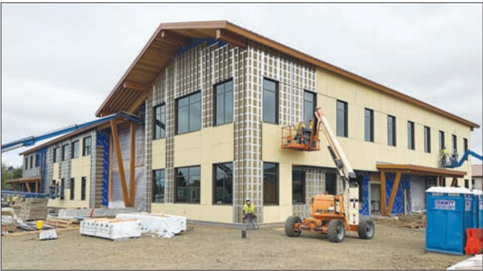
Tiling being installed on the new healthcare education building's exterior that will be painted to match the main building.
