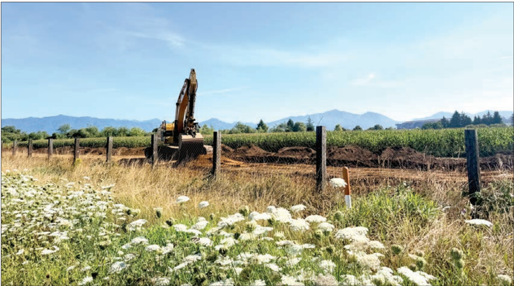
An excavator at work on a section of the pipe along Highway 101.
