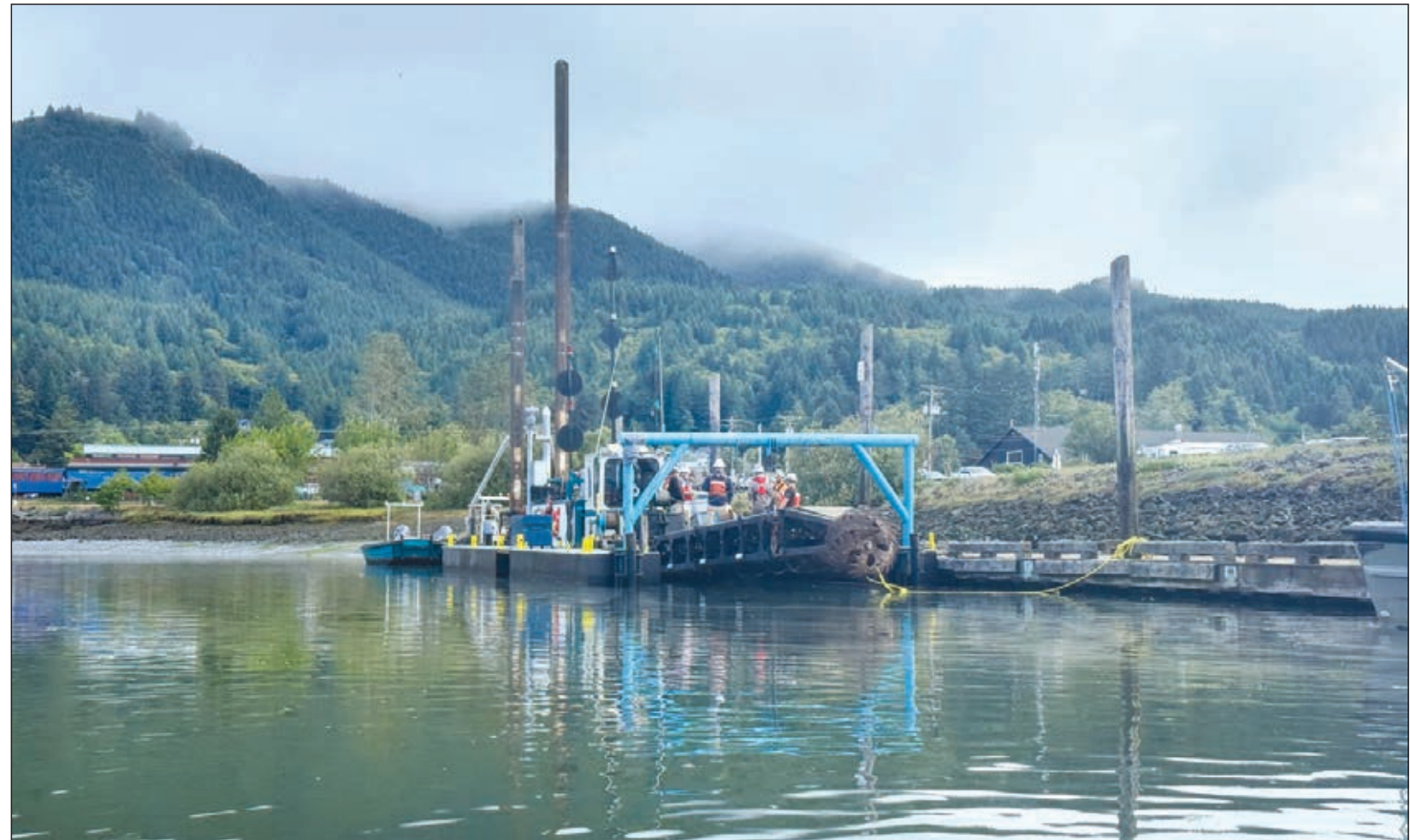
One of the dredging barges that will be used in the boat basin at the Port of Garibaldi sits at the transient dock in the port awaiting deployment.
