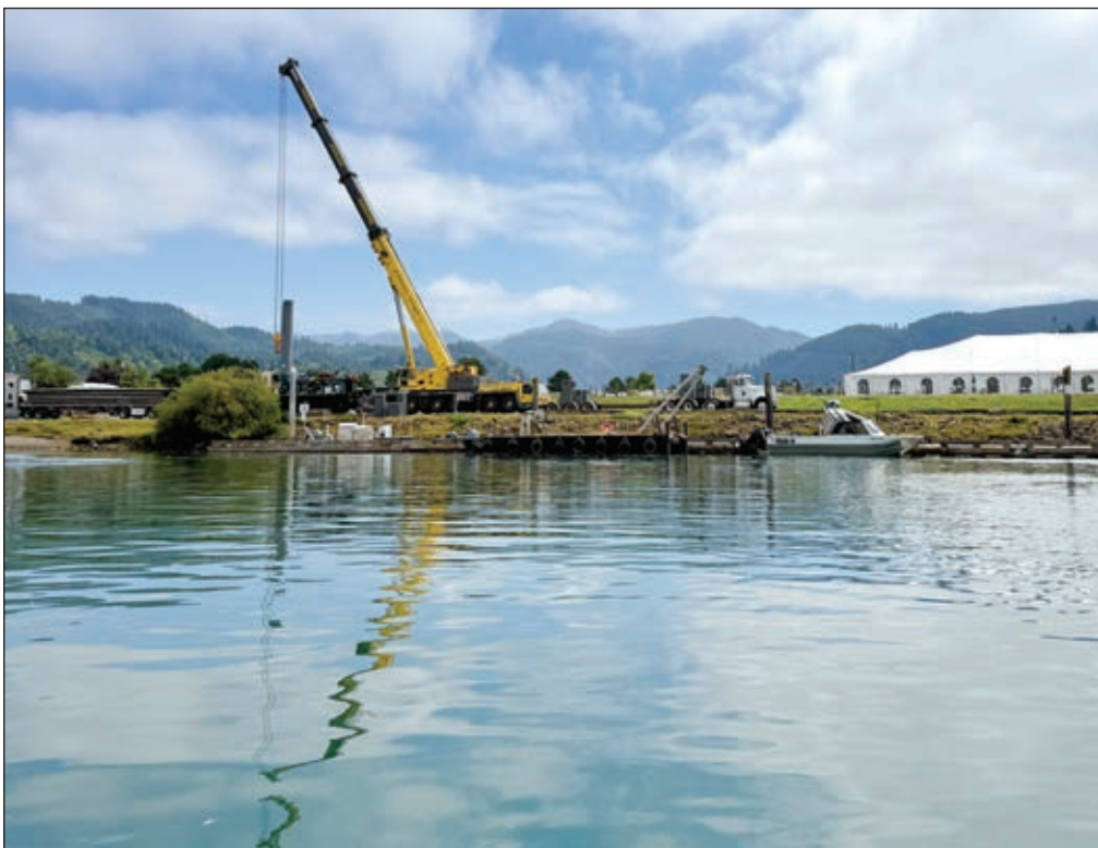
A crane unloads pipe that will be used in the project during the first week of August.
