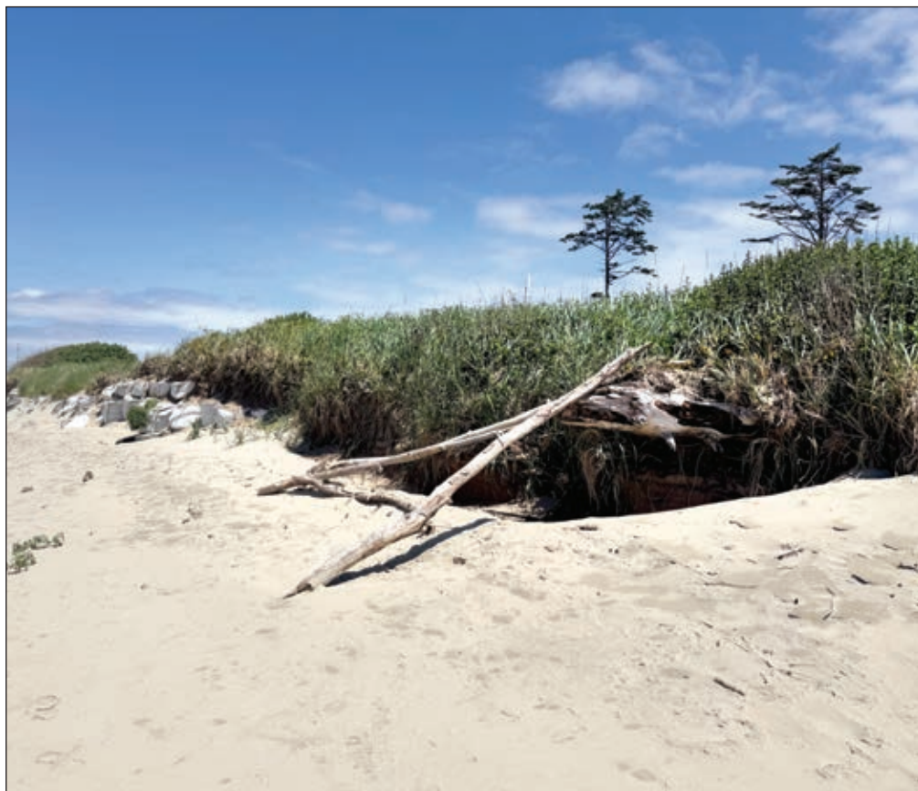
A section of the manmade dune that will be repaired this summer and fall to prevent flooding in the A and B campsite loops.
