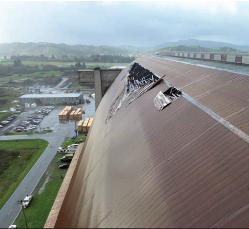
PHOTO COURTESY STIMSON LUMBER The damaged area of the building’s roof as viewed during a drone flight the day after the windstorm.
