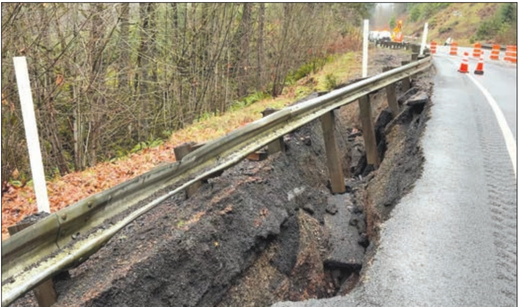
The landslide caused significant damage to the road's shoulder as well.
