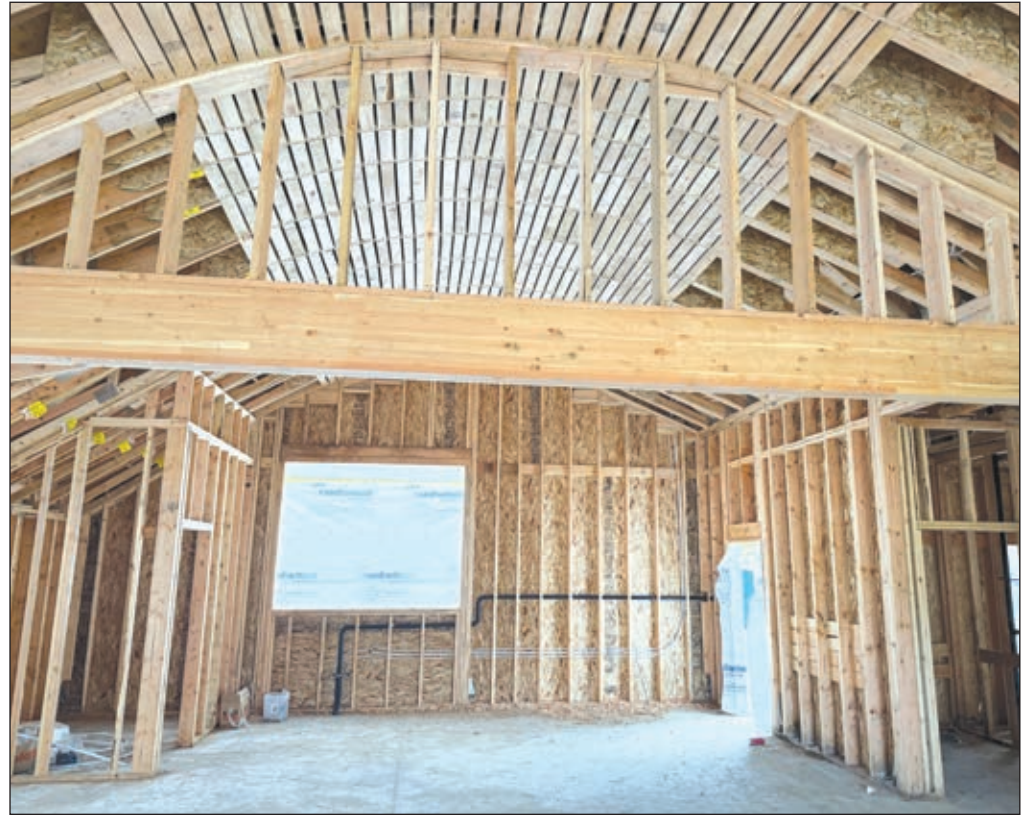
The community gathering room's interior in the clubhouse features an arched ceiling.
