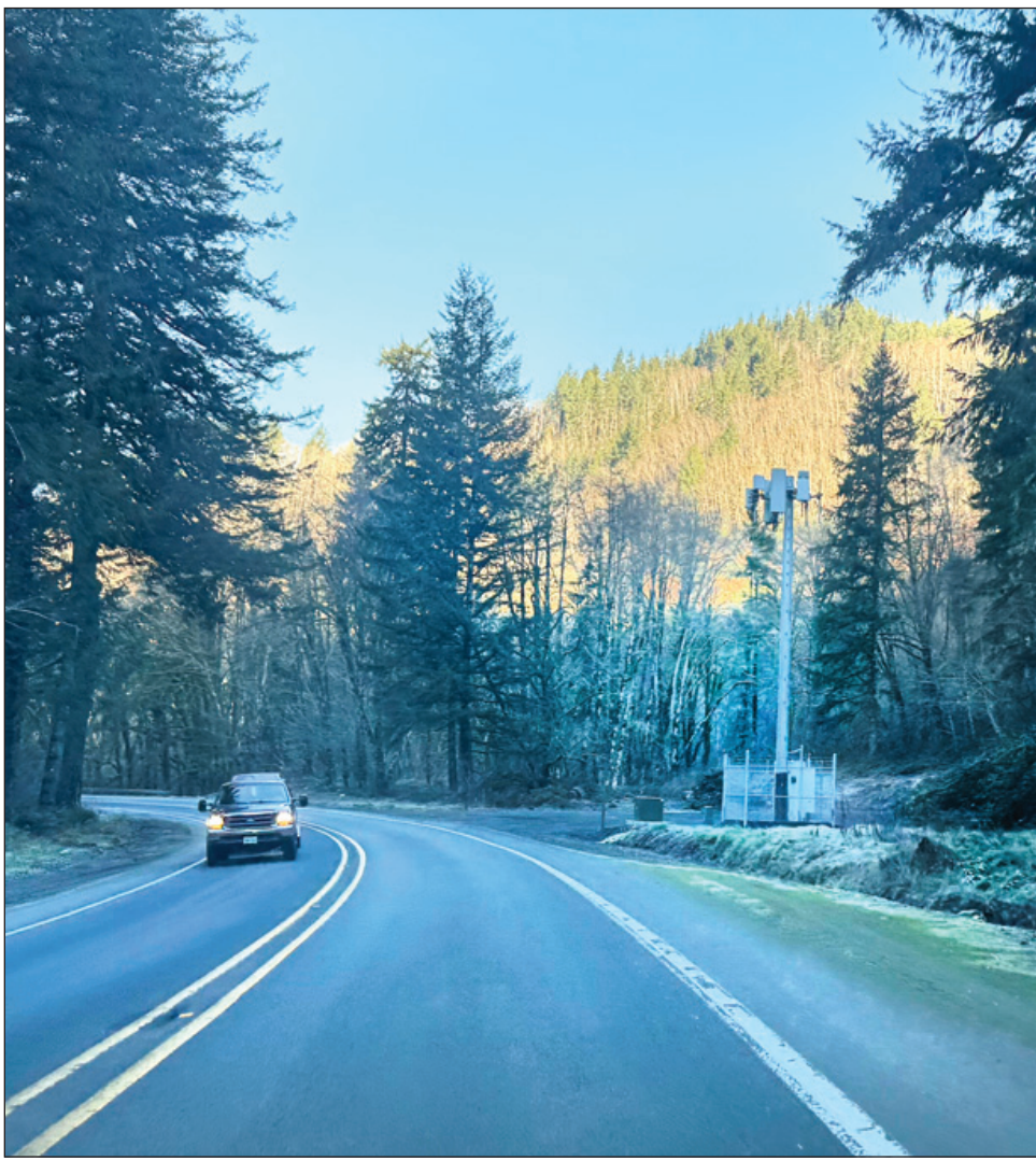
One of the new 5G towers beside Highway 6.
