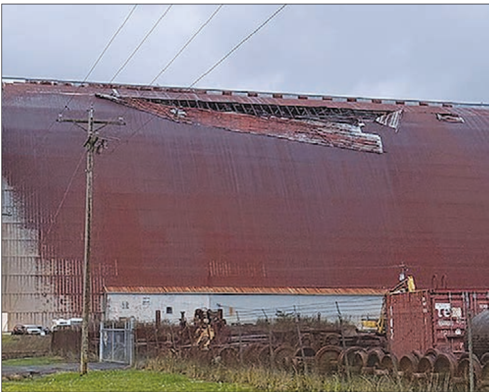
A windstorm caused a hole in the roof of Hangar B at the port of Tillamook Bay. Hangar B is closed indefinitely as a fix is determined. Photos courtesy Port of Tillamook Bay
