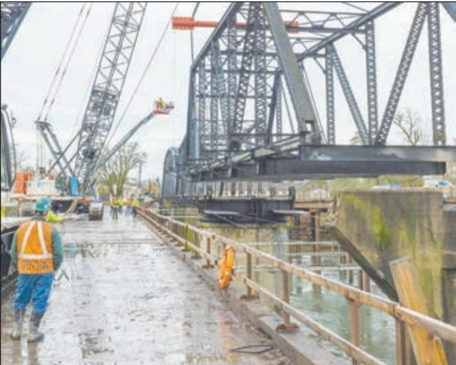
Courtesy photo from ODOT Construction crews use a crane to remove the old Van Buren Bridge in Corvallis in preparation for the new bridge.
