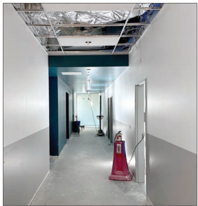
The clinic's interior awaits flooring and ceiling installation.
