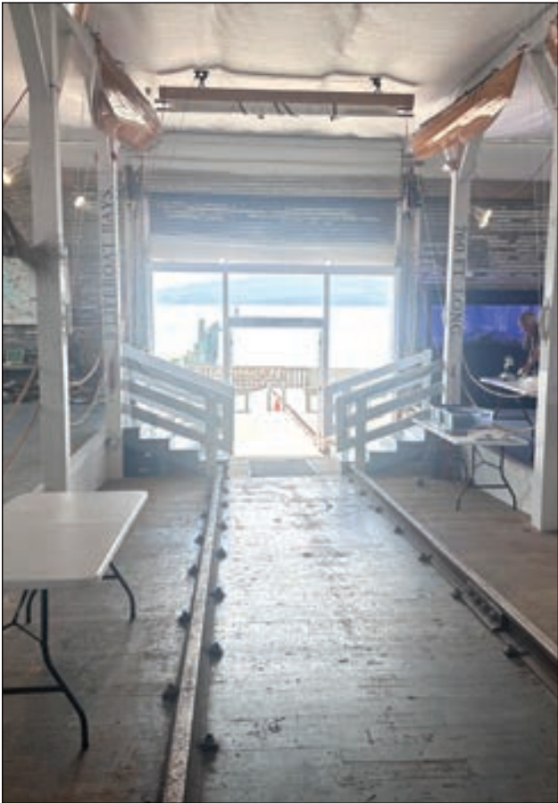
The interior of the boathouse, with one of the sets of rails used for lowering boats into the water visible in the middle bay.
