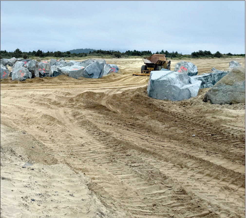
A rock truck at work grading the largely empty sandy area near the jetty that served as a stockpiling area for rocks throughout the project.
