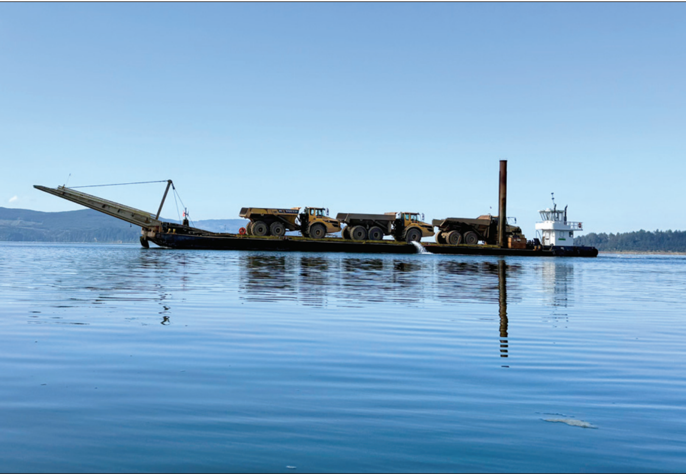
Three rock trucks return from Kincheloe Point to the Port of Garibaldi after depositing stones at the work site on a sunnier day this summer.
