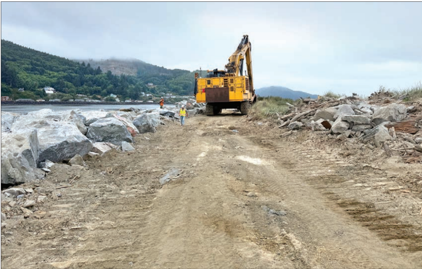
An excavator at work rearranging stones in a section of jetty near the root with which Guymon was not completely satisfied.
