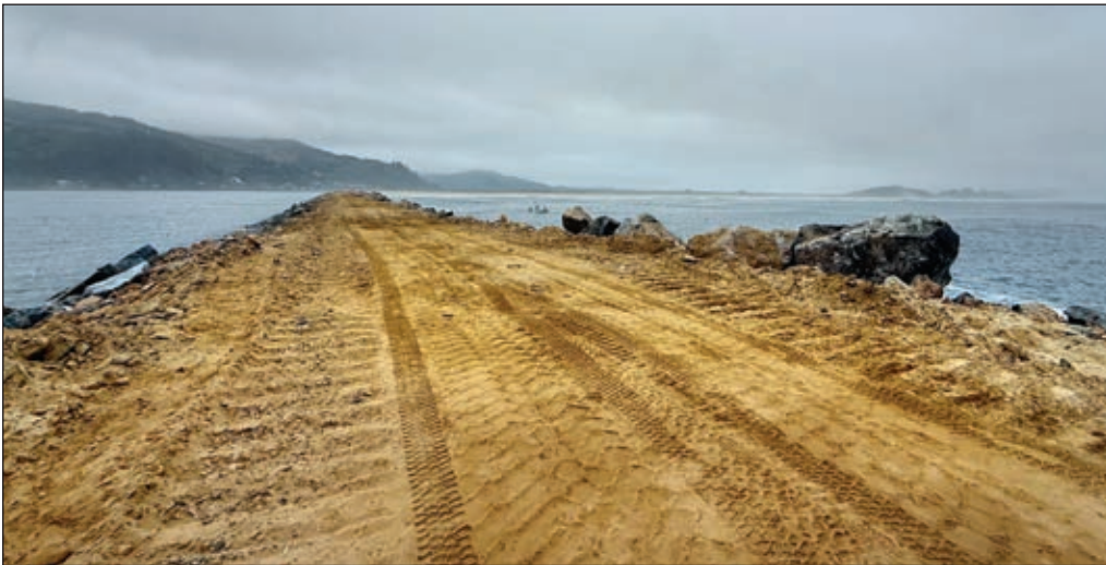
The haul road atop the south jetty that has been used the last two summers by rock trucks to access its head.
