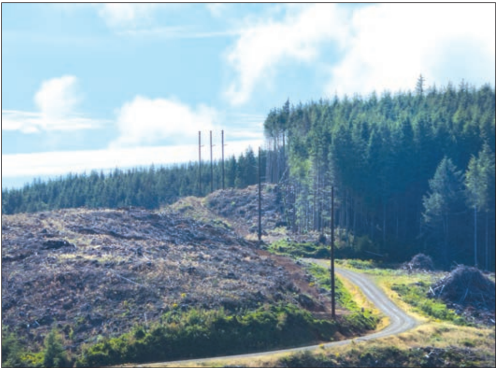
Views of poles along the route as it crosses Mount Maxwell. Courtesy TPUC
