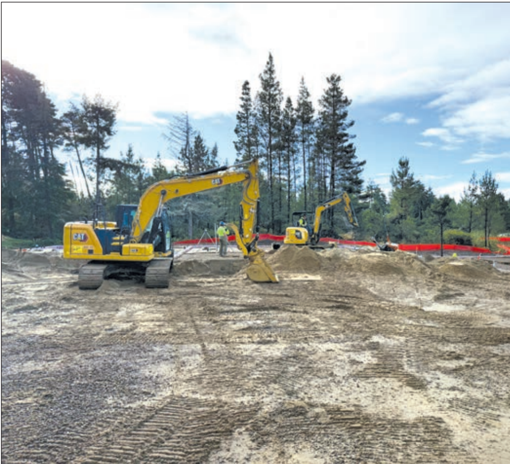
Workers prepare for the concrete slab bases of the five apartment buildings and community center to be poured.
