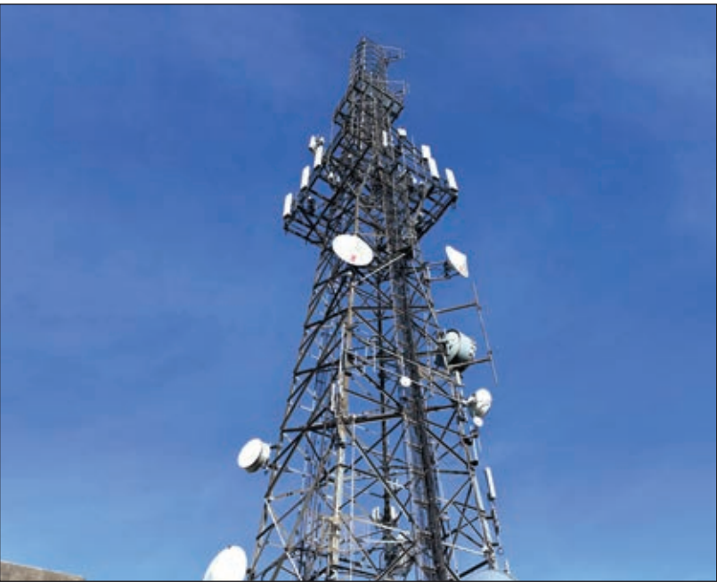
WILL CHAPPELL / COUNTRY MEDIA, INC. The tower on top of Cape Meares that hosts transmitters for the county's emergency radio system, as well as a plethora of other broadcast, cellular and amateur and professional radio equipment. In addition to sometimes competing for frequencies, the large number of loose cables left by past users cause literal noise on radios as they move in the wind.
