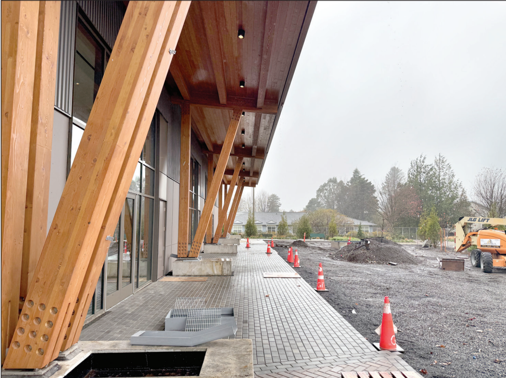
Events in the new community room will be able to spill onto the plaza.
