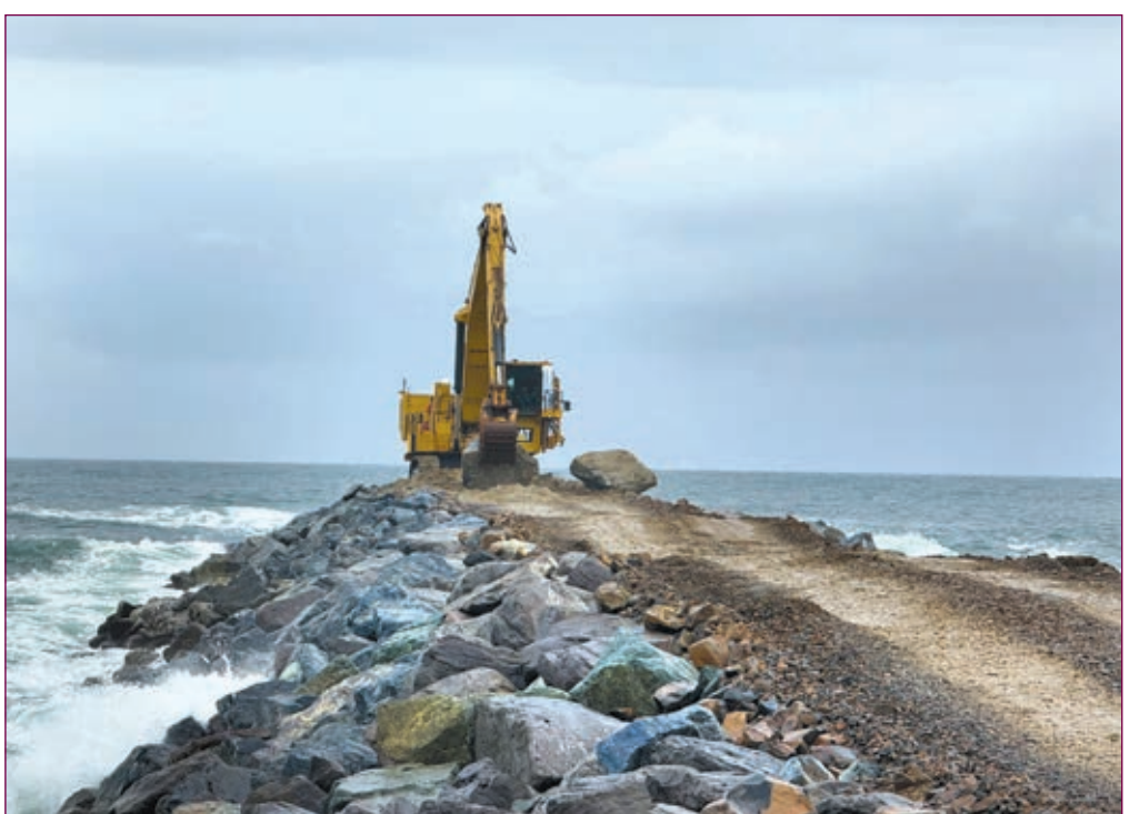
The excavator picking up a rock for use in the head.
