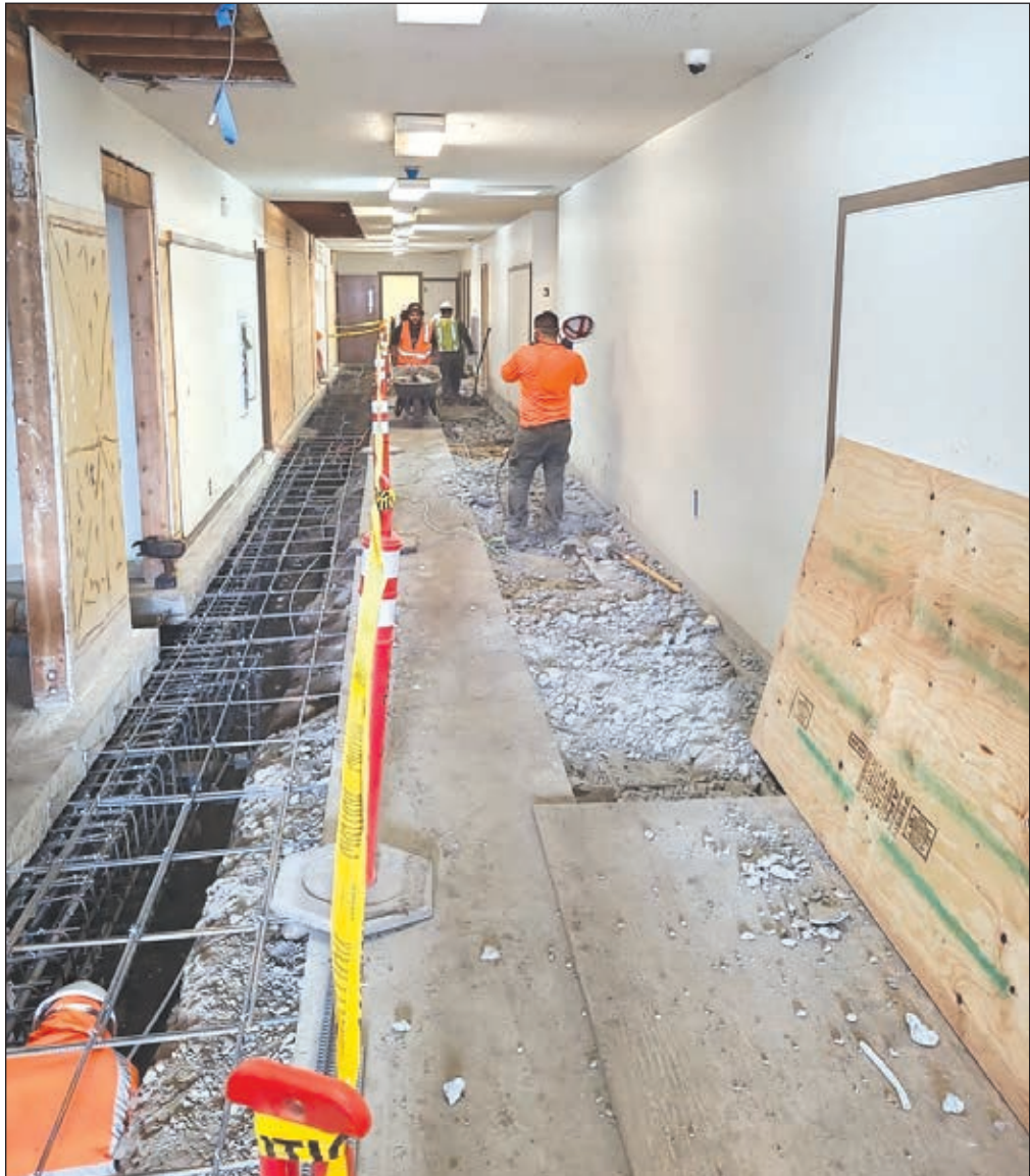
Seismic resiliency work in Liberty Elementary School this summer included adding a seismic isolation gap. Photo courtesy Tillamook School District
