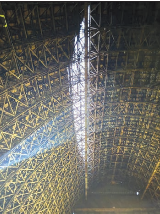
A windstorm caused a hole in the roof of Hangar B at the port of Tillamook Bay.
