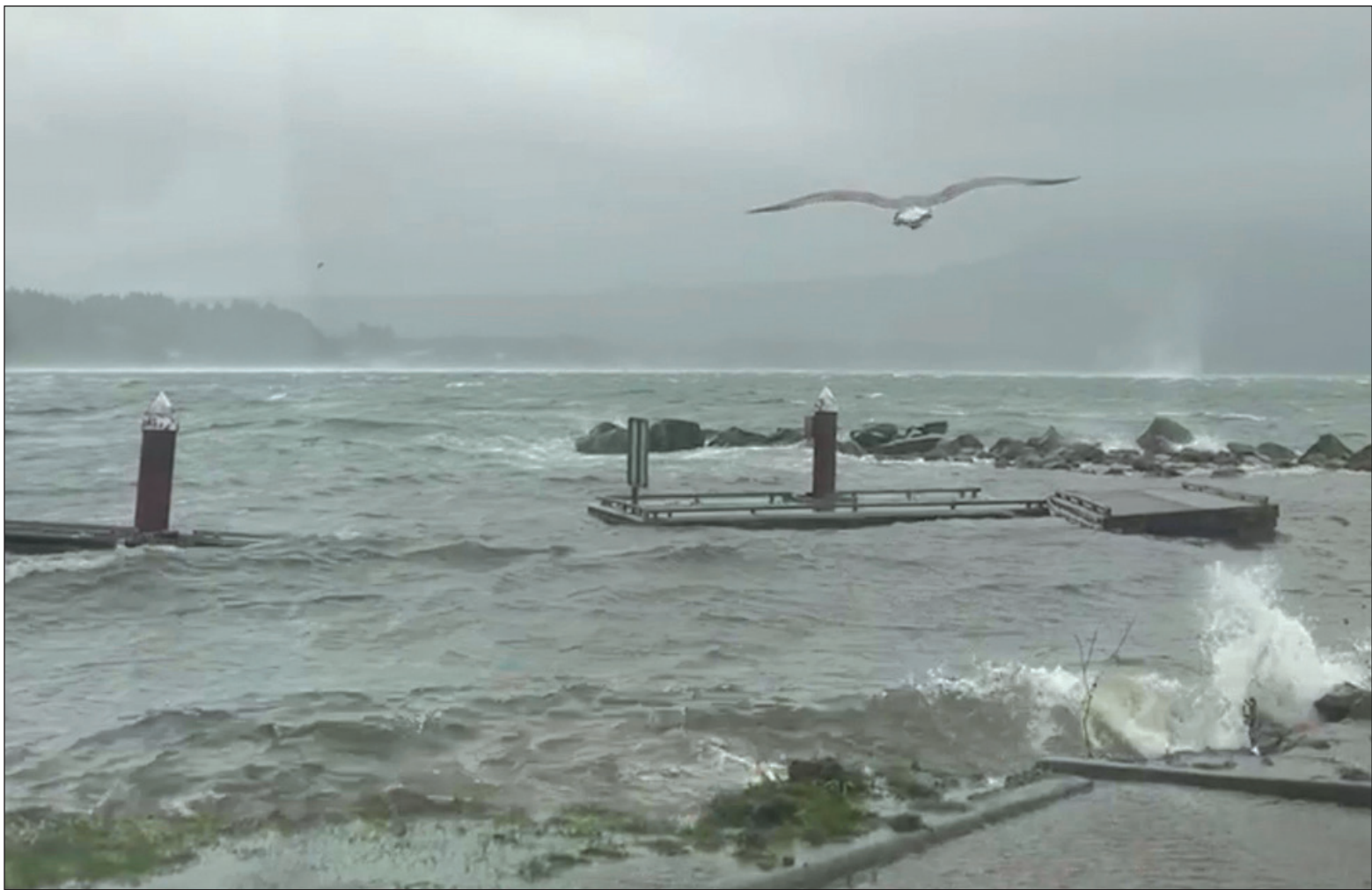
The dock at the Tillamook County boat launch in Netarts had taken significant damage, including several sections blown away, by high tide around noon on November 6.
