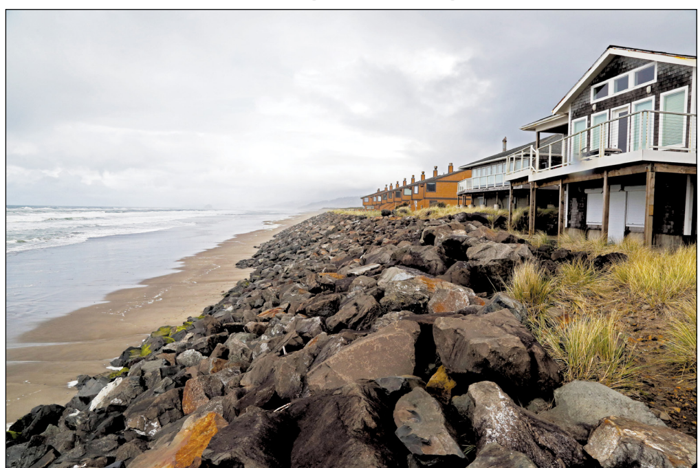
Oceanfront landowners in Neskowin use rock revetments, or rip-rap, to protect their properties from erosion. The decision has implications for public access and recreation.
