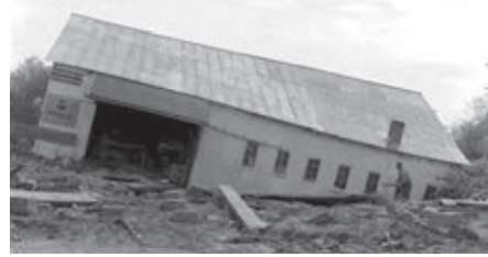
This feed store "fell in" when its owners were moving it across Ferry Creek. The building is to the east of Grand Avenue today.
