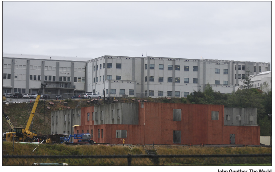
John Gunther, The World The different colors of the pre-cast panels used for the new Marshfield Junior High School are shown by this photo taken from a nearby street.
