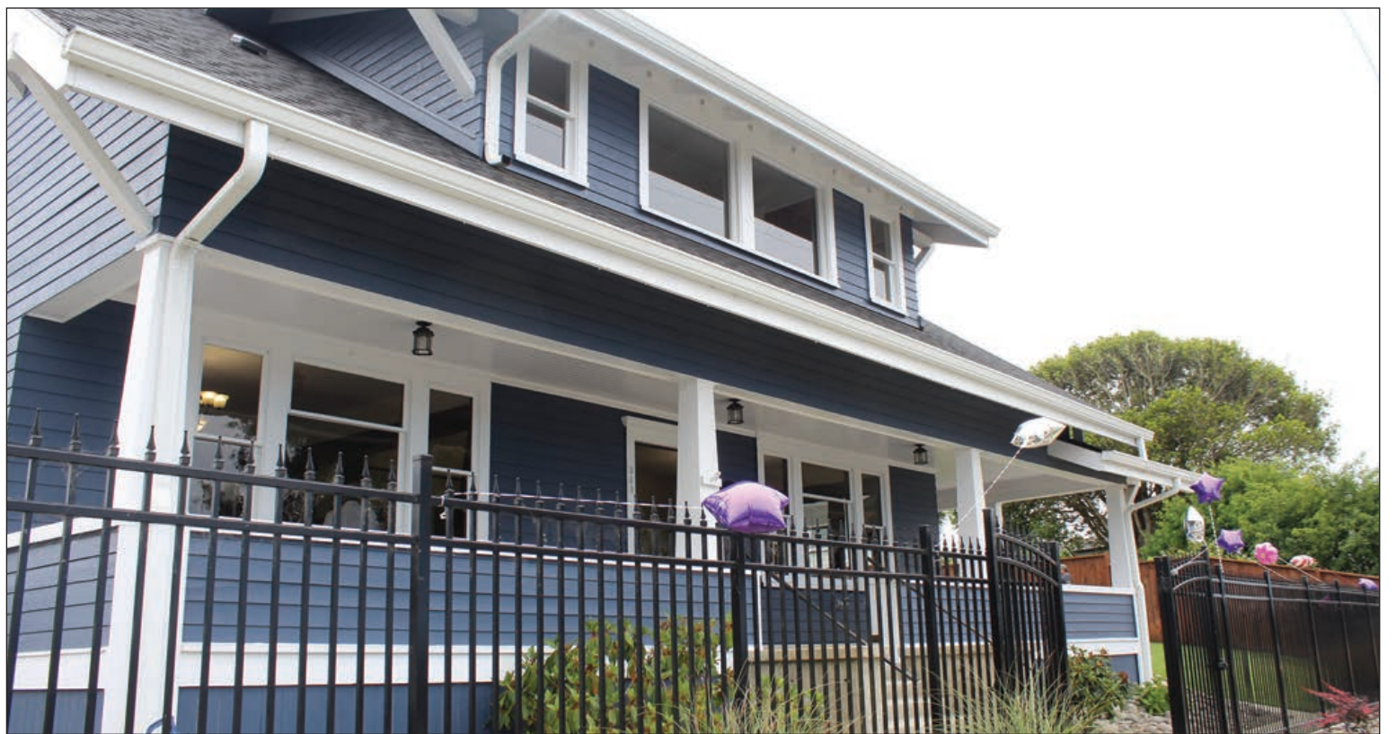
Photos by David Rupkalvis/The World The Blue House on Cape Arago Highway has been updated with the newest technology while maintaining as much of its original character as possible. During construction, Wayne Schrunk kept the original wood for the floors, stairs and much of the walls.
