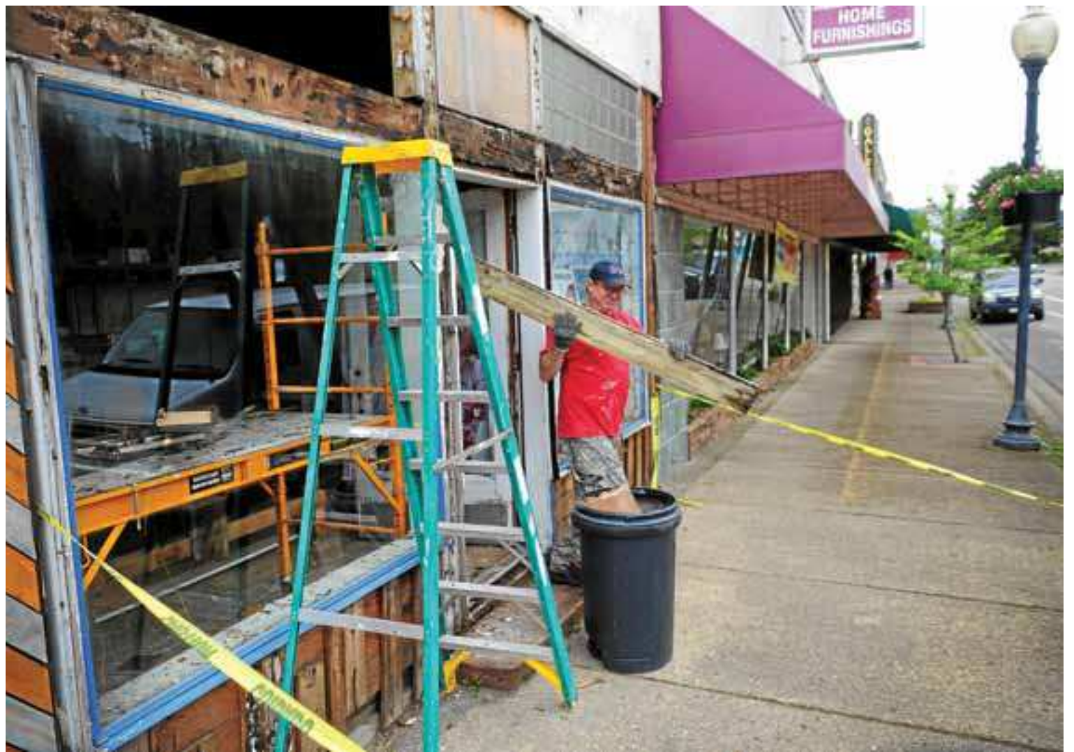
Tommy Starner, an owner of Butterfly Effect in Reedsport, repairs part of the business facade earlier this spring.
